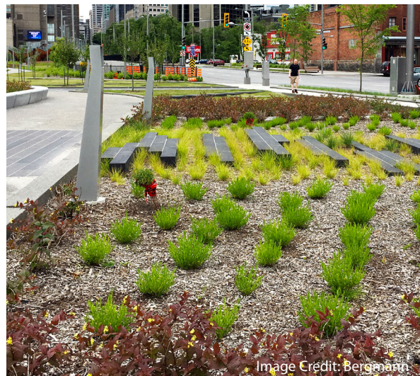
Rain Gardens Enhance Urban Sites. This example demonstrates how stormwater management can be an integral part of site design. A large rain garden not only stores, filters, and infiltrates stormwater, but provides opportunities for public interaction, art, and streetscape beautification.
