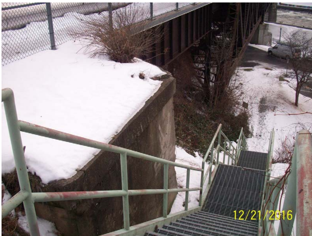
Photo 6 – Wingwall and stairs at north side of abutment
