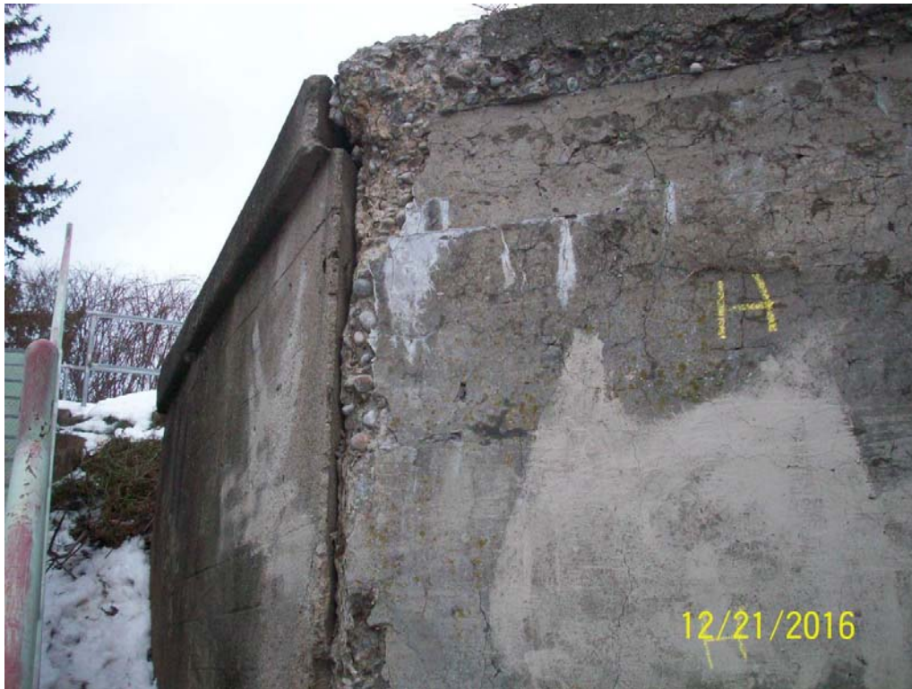
Photo 7 – Separation at north wingwall construction joint
