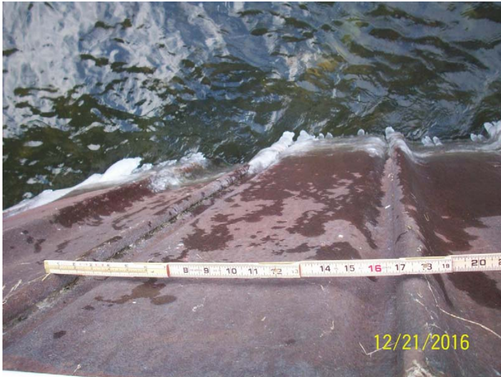
Photo 5 – Top of typical cellular wall pile, 1 st cell near STA 20 shown.
