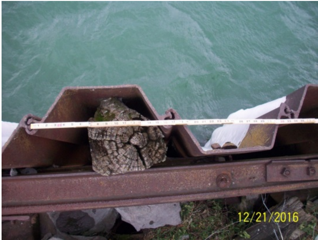
Photo 33 – Top of typical sheet pile, at northwest corner of pier
