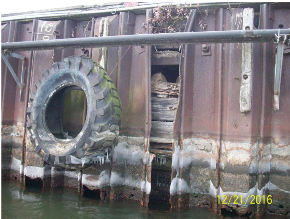
Photo 22 - Sheet pile wall, missing section of pile exposed timber cribbing at STA 425
