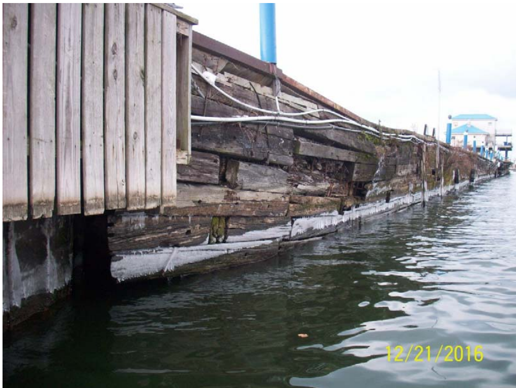
Photo 8 – Timber cribbing wall, beginning at STA 129
