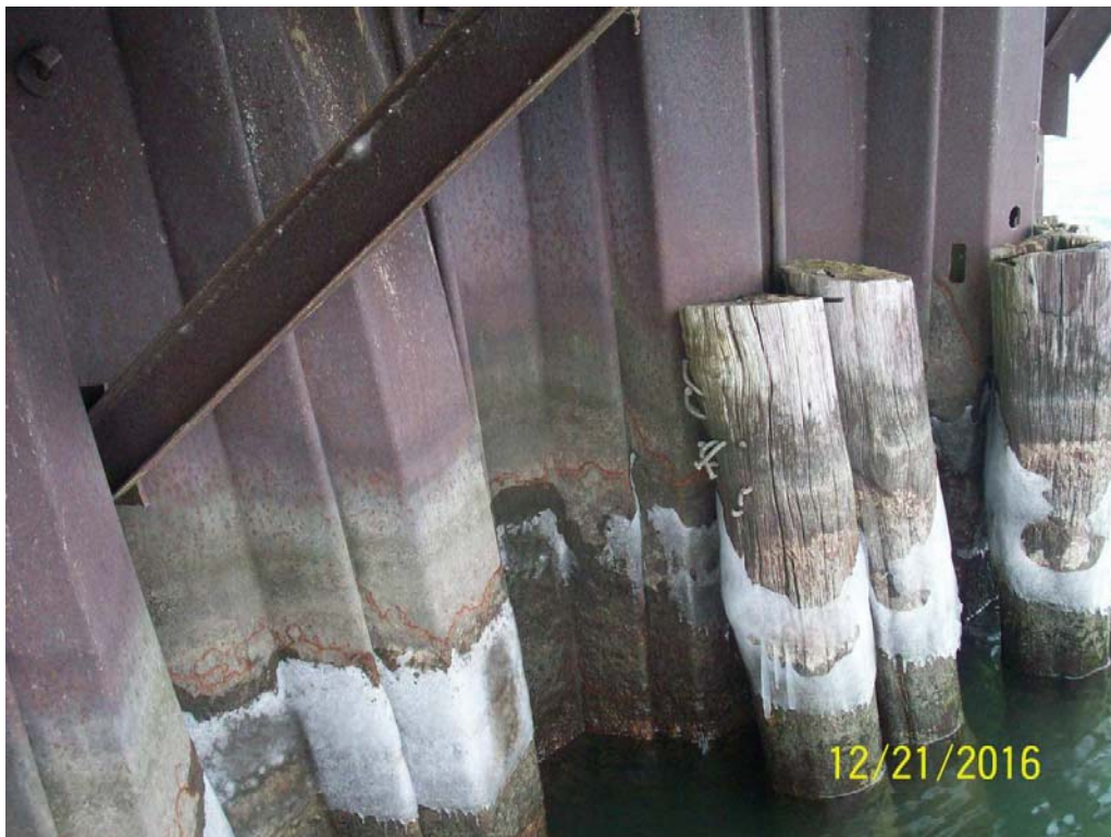
Photo 30 – Sheet pile wall and timber piles at STA 850
