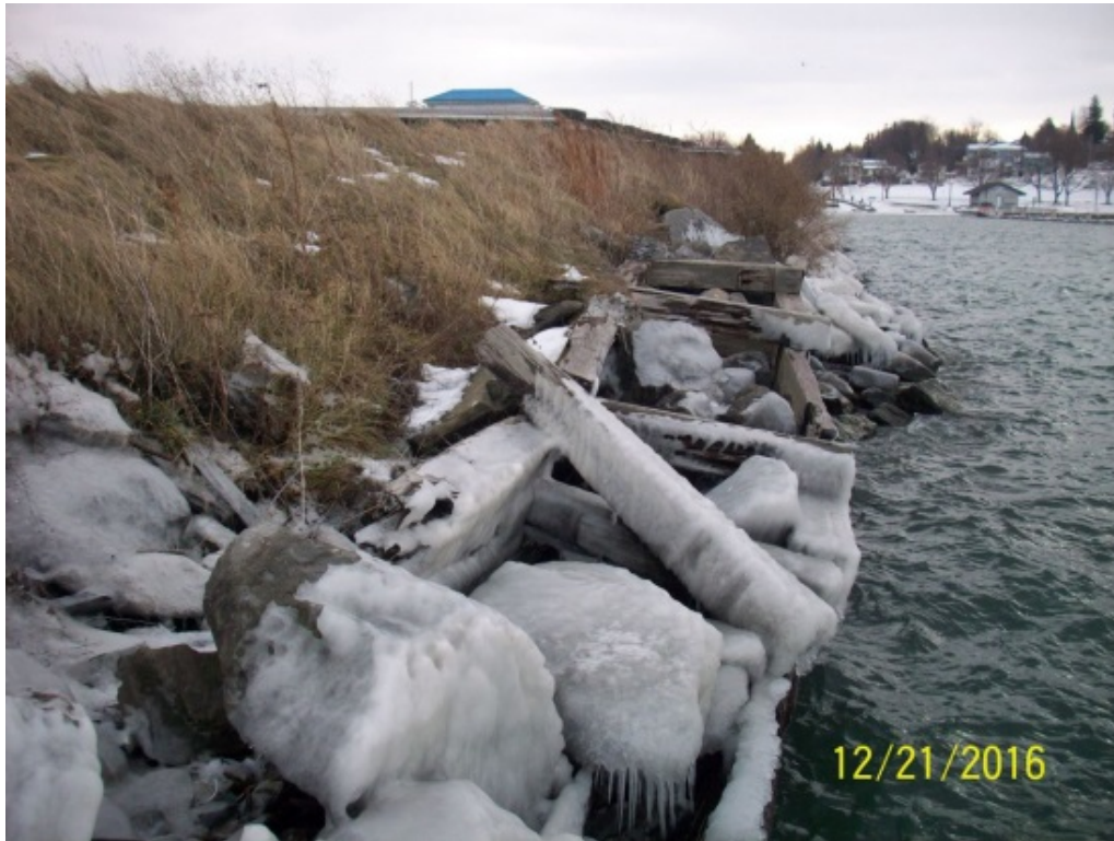
Photo 39 – Remnants of timber cribbing at near northwest corner of pier
