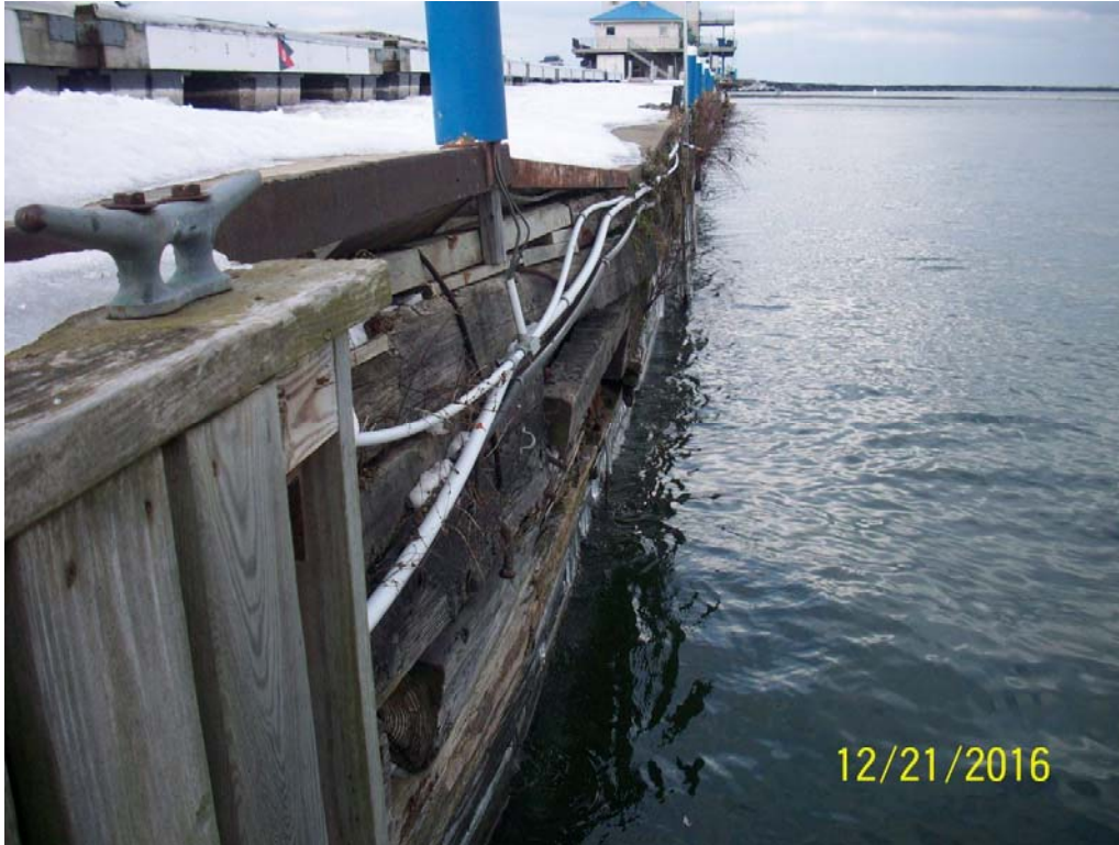
Photo 13 – Top of timber cribbing wall, showing settlement between STA 135 and 160
