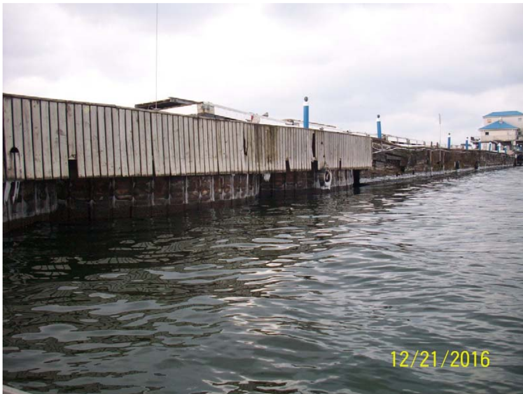
Photo 4 - Cellular sheet pile wall near STA 80
