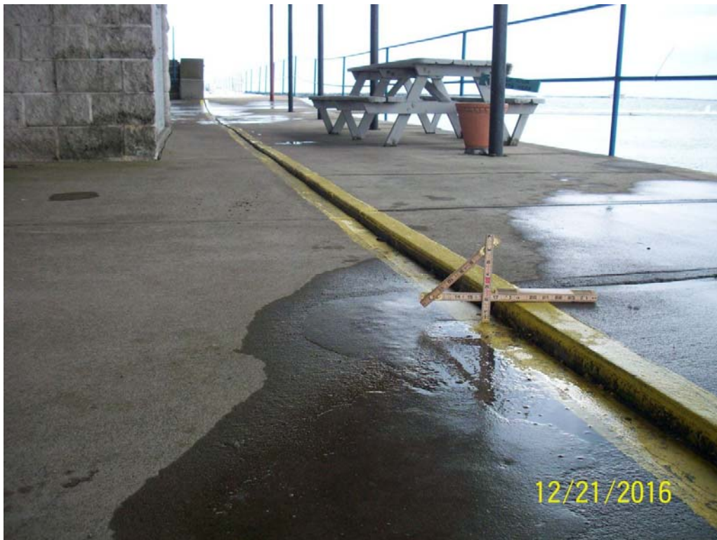
Photo 38 – Settlement of concrete slab behind sheet pile wall near STA 500
