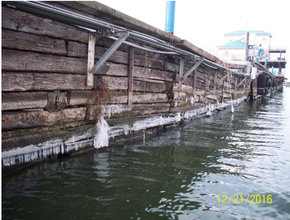
Photo 11 - Timber cribbing wall, looking north near STA 300
