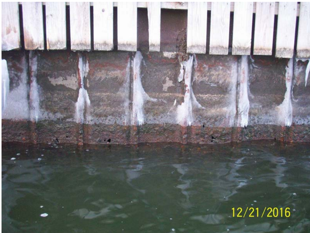
Photo 6 – Cellular wall near STA 120, showing typical corrosion near water level
