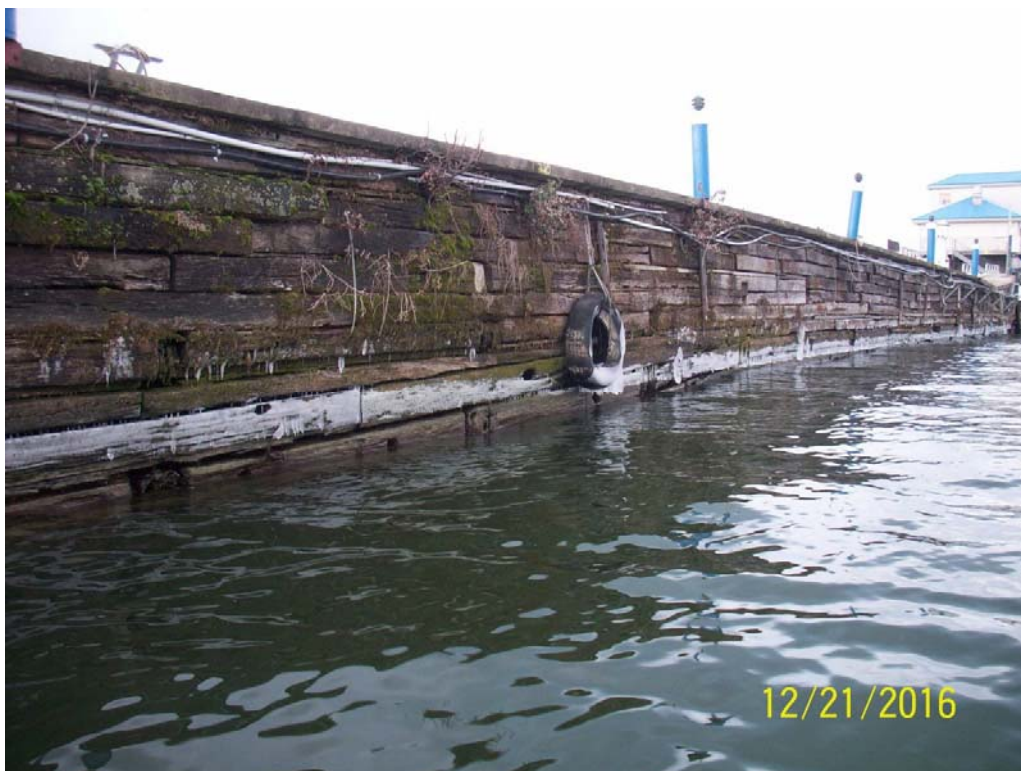
Photo 10 - Timber cribbing wall, looking north near STA 200
