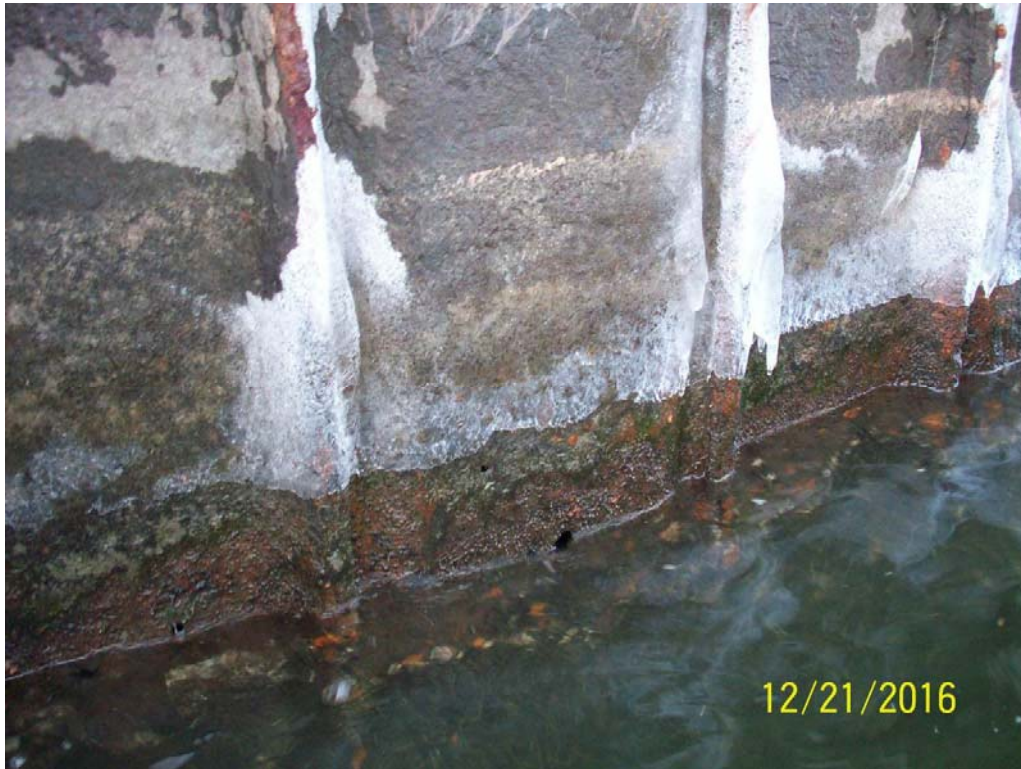
Photo 7 - Cellular wall near STA 120, close-up of typical pile corrosion
