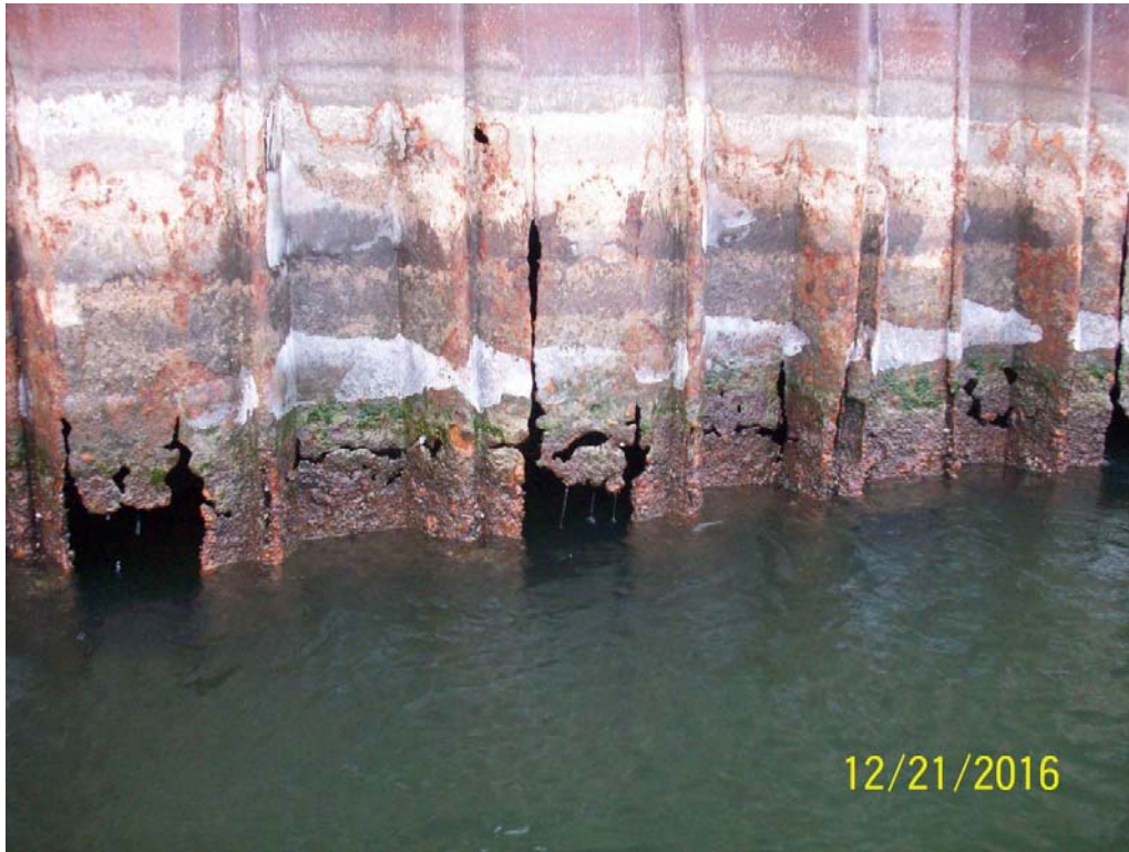
Photo 23 - Sheet pile wall, close-up of typical holes near low water level at STA 600
