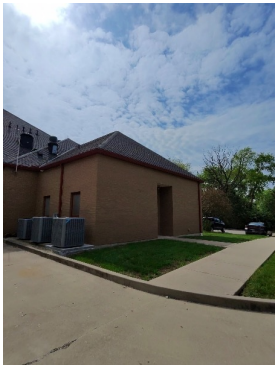
Exterior of Building
