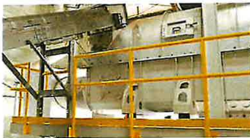
5: If the glass is wet, it is sent through a fluidized bed dryer to remove moisture.
