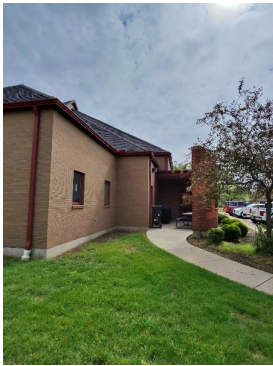
Exterior of Building
