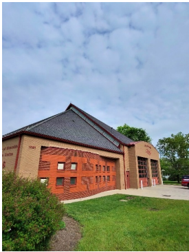
Exterior of Building
