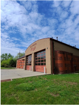
Exterior of Building
