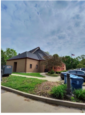
Exterior of Building
