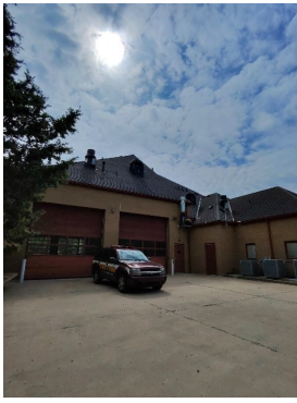
Exterior of Building
