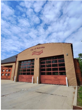
Exterior of Building
