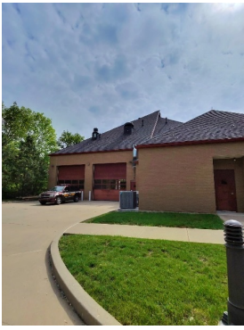
Exterior of Building
