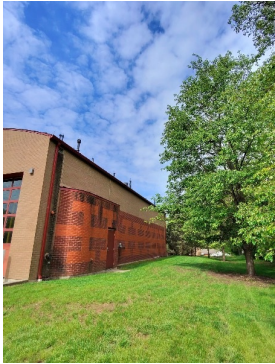
Exterior of Building
