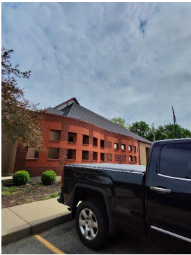
Exterior of Building
