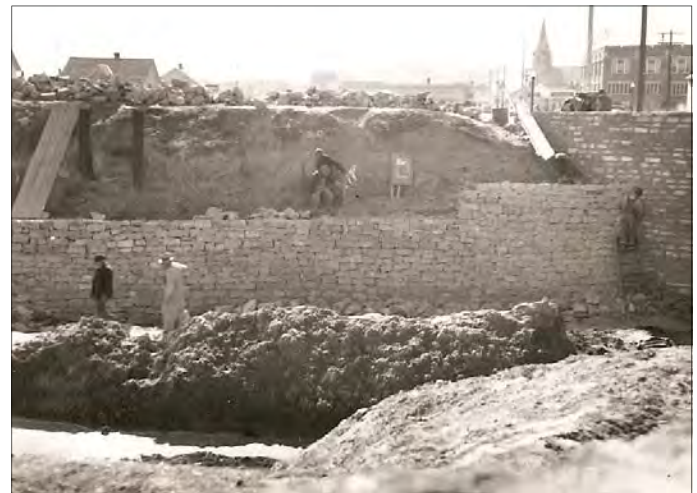
Works Progress Administration construction of retaining wall along Bitter Creek, 1941.
