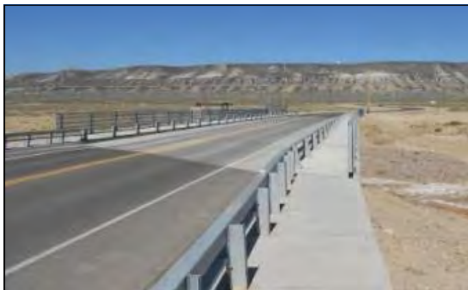
Industrial Drive Extension, Completed 2012.
