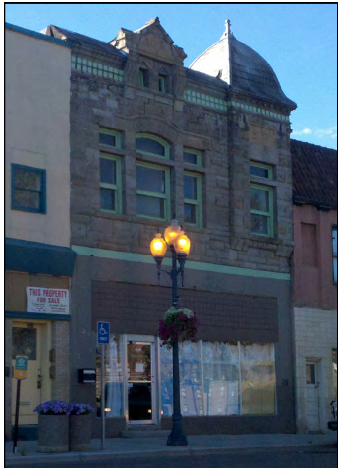
Historically Contributing Building on South Main Street.
