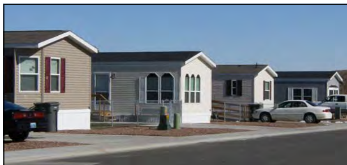
Aspen Village Mobile Home Park, Constructed 2007.
