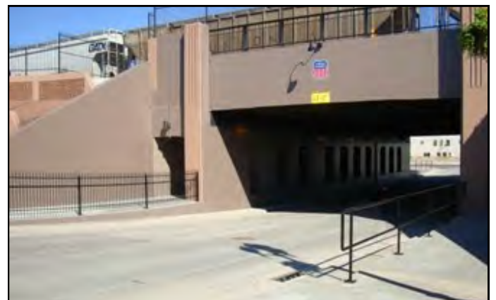
Figure 6.10: Recently Renovated M Street Vehicular/Pedestrian Underpass.
