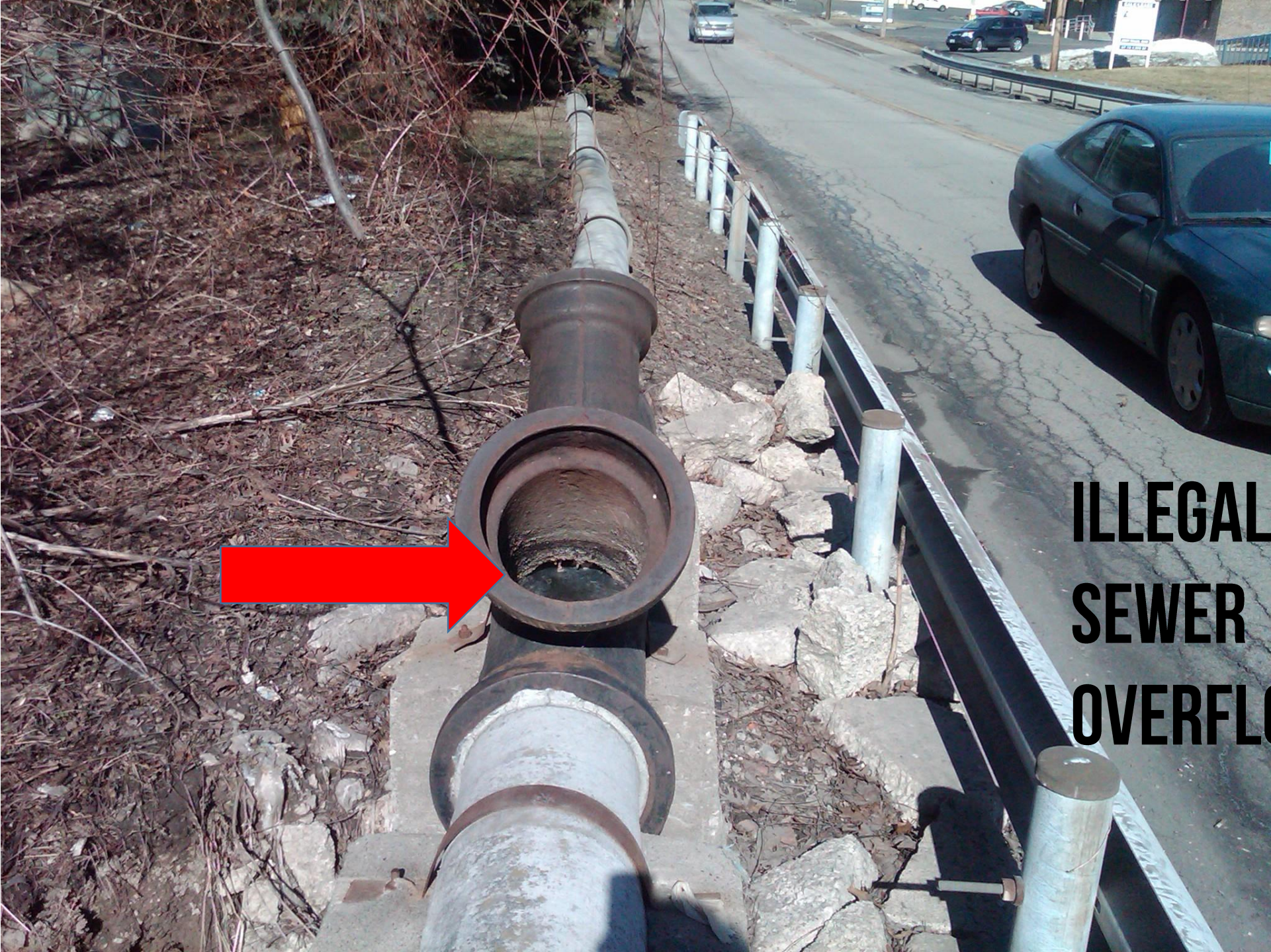
Illegal sanitary sewer overflow along Dixie Highway, January 2011.
