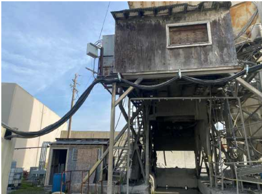
Photo 6: View of non-operable batch plant and air compressor room, facing northeast.
