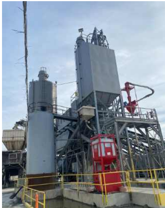
Photo 4: View of operational batch plant, facing east.
