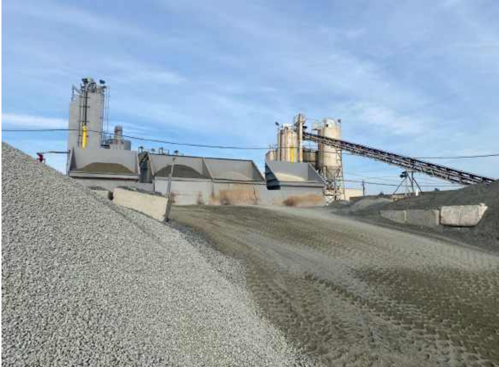
Photo 13: View of dry materials storage area, facing north.
