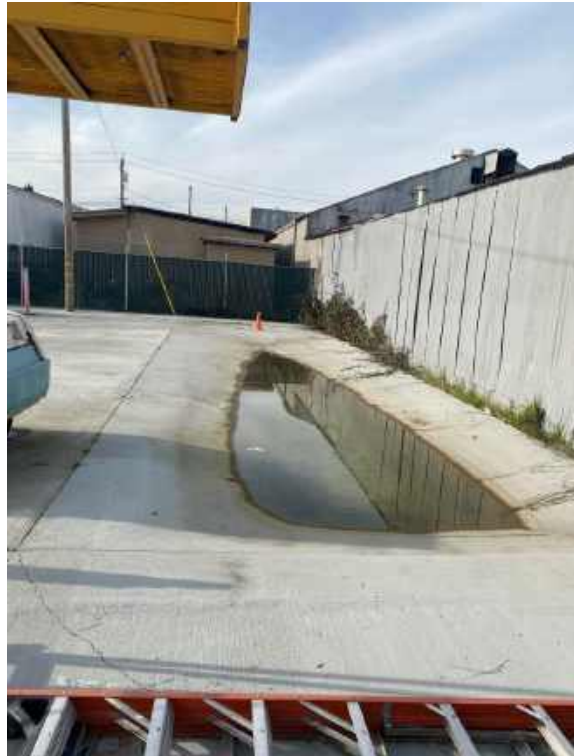
Photo 5: View of stormwater swale, facing southwest.
