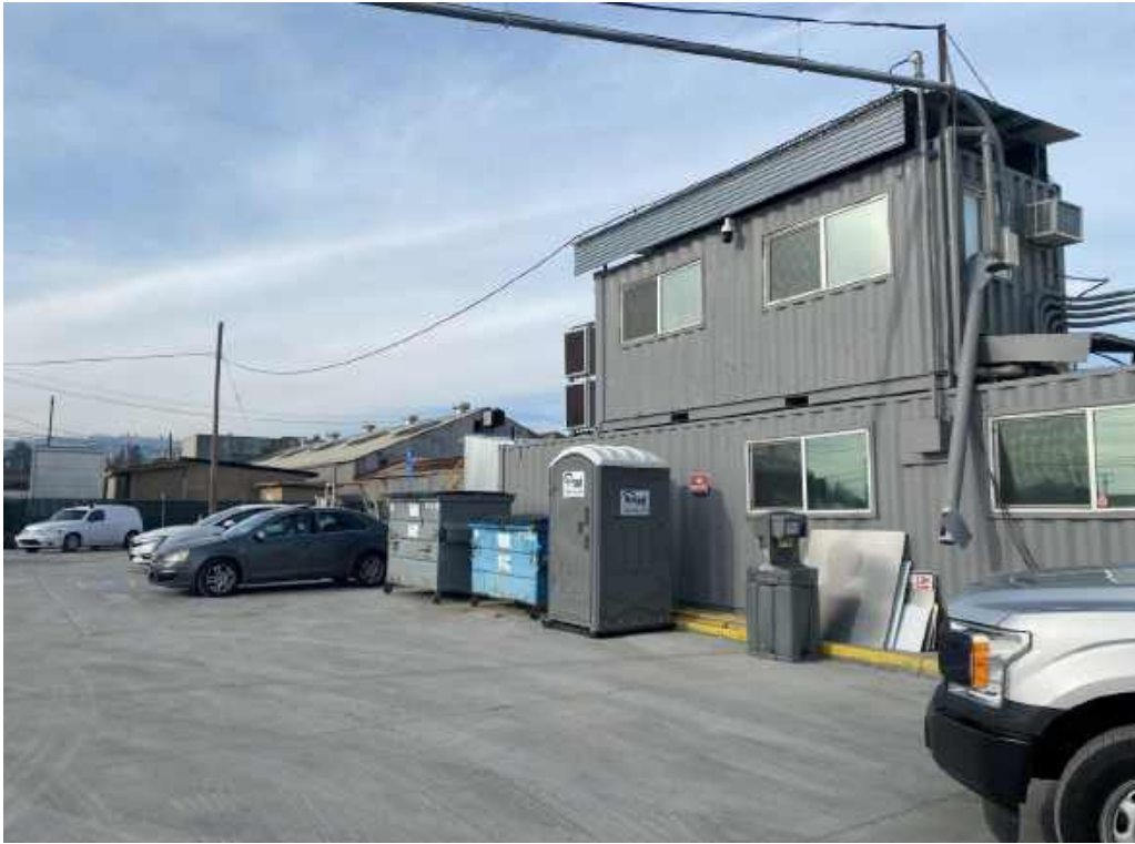
Photo 3: View of office building and control room, facing west.
