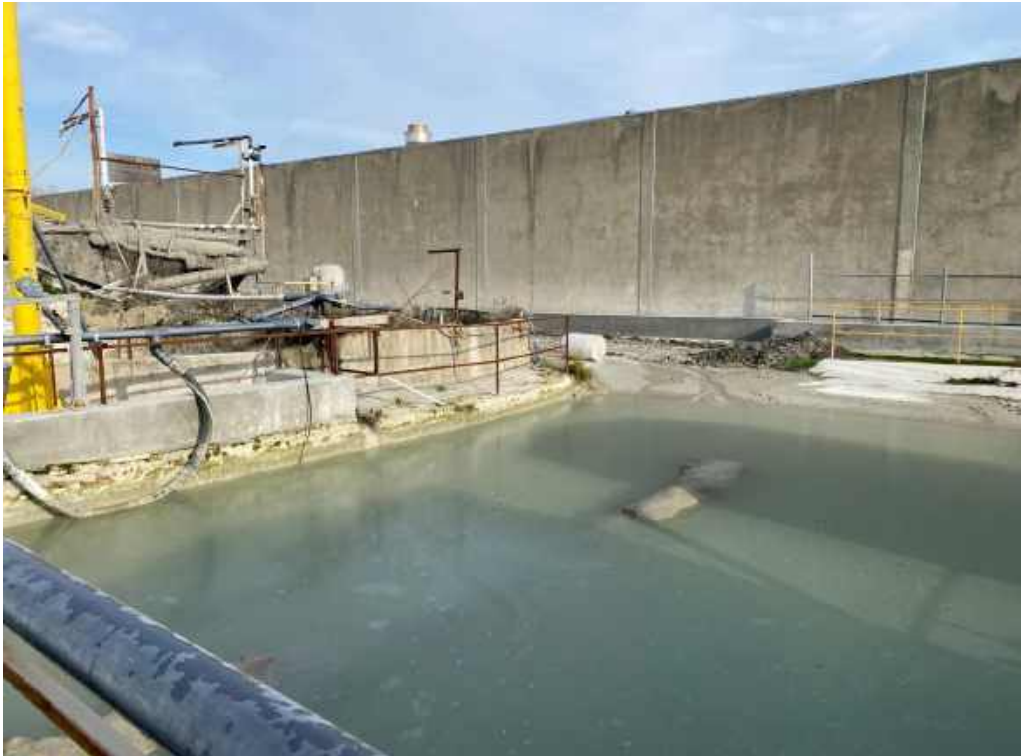
Photo 11: View of the main reclamation pond, facing northeast.
