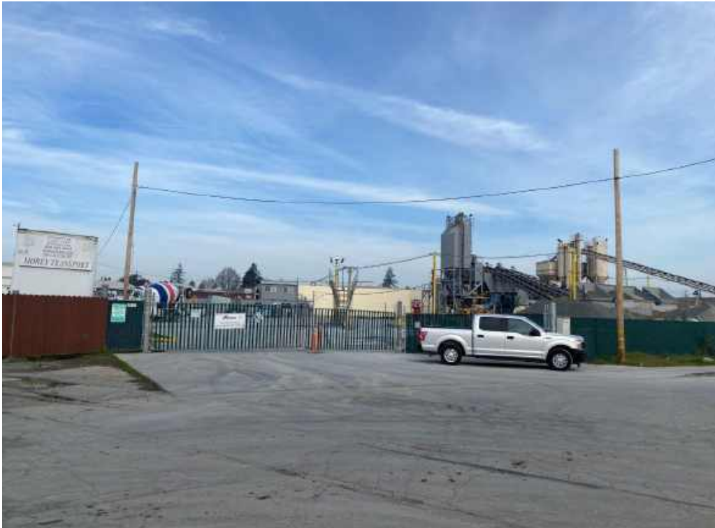
Photo 1: View of the entrance to the CEMEX facility at 1026 Bransten Road, facing north.
