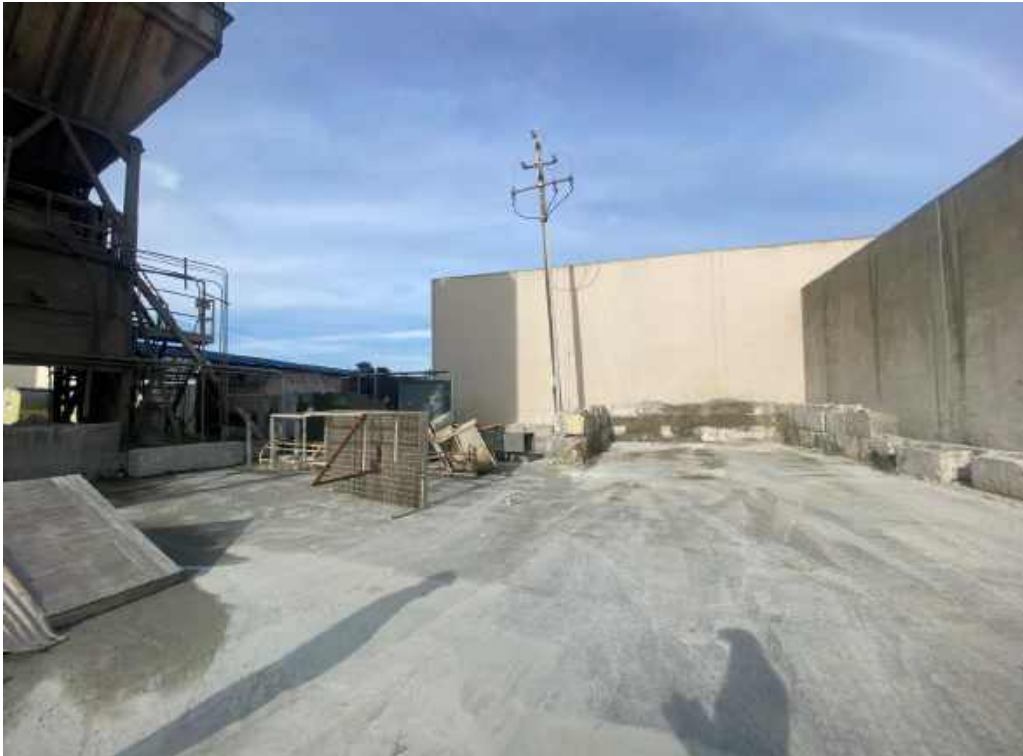
Photo 9: View of the retaining wall which captures stormwater runoff, facing northwest.
