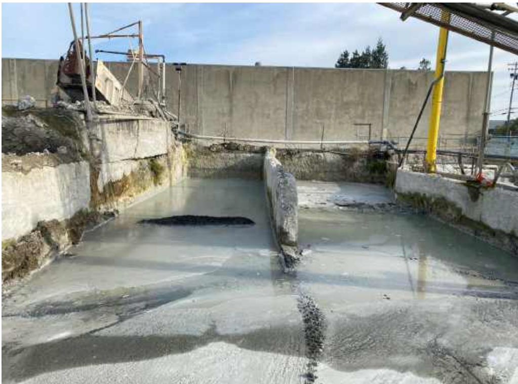
Photo 10: View of the first two weirs of the reclamation pond system, facing northeast.
