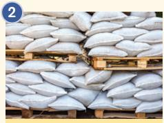
**Close** each bag by folding over the top. Tying bags tightly closed can cause gaps to open up in your wall.
