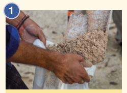
**Fill** each sandbag only to the fill line (or about halfway). Filling the bags all the way up is actually counter-productive, and causes the bags to be less efficient at keeping water out.
