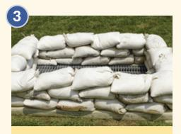
**Lay** the bags flat and horizontally on top of each other, as if you were laying bricks. Let gravity do the work to press the bags together.
