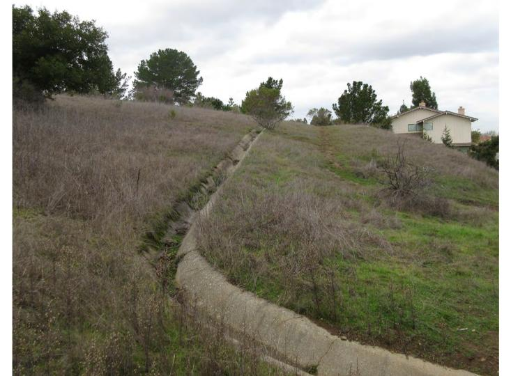
10 CONCRETE DRAINAGE CHANNEL
