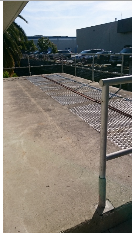
Figure 2. Confined space vaults screen and guardrails to prevent fall to lower level water channel. Use concrete anchors when work requires removal of guardrails. Do not use guardrails as fall protection anchors.
