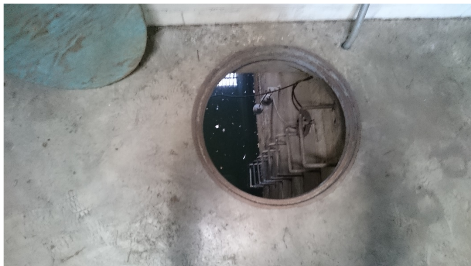
Figure 1. Confined space access to lower level wet well. Employees do not use fixed ladder.
