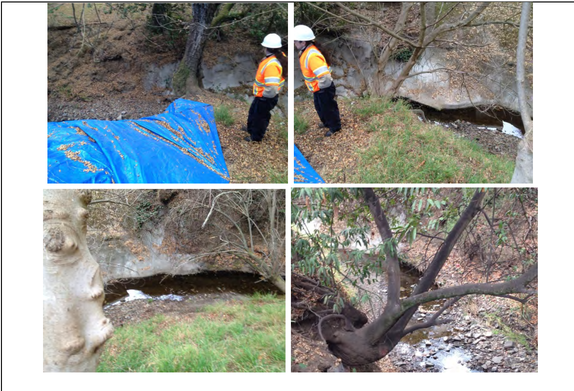
Photo 25. Taken from approximately 1,860 ft upstream of the culvert crossing at Chula Vista Drive facing the left bank beginning upstream of the cut bank and moving downstream, respectively
