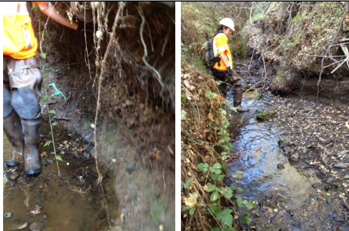
Photo 14. Taken approximately 840 ft upstream of the Live Oak culvert facing the left bank and upstream, respectively
