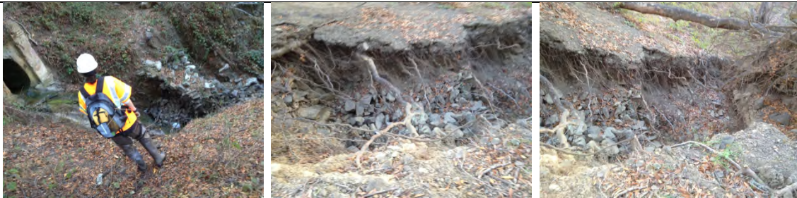
Photo 6. Taken approximately 2,000 ft upstream of the Live Oak culvert at the low flow outfall of Water Dog Lake facing upstream, left bank, and downstream, respectively
