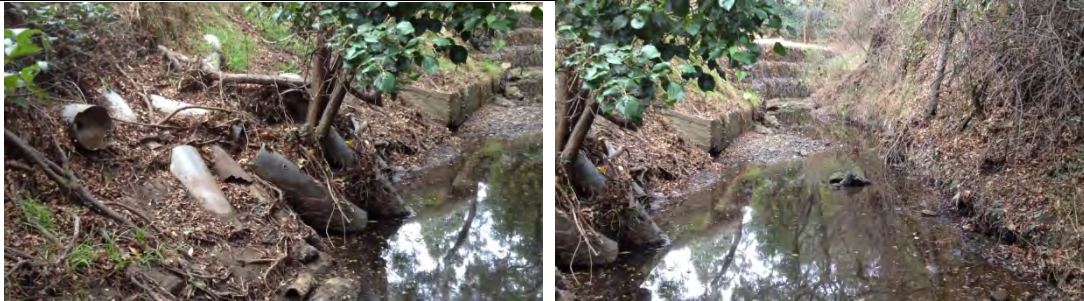
Photo 31. Taken approximately 700 ft upstream of the culvert crossing at Chula Vista Drive facing upstream and downstream, respectively
