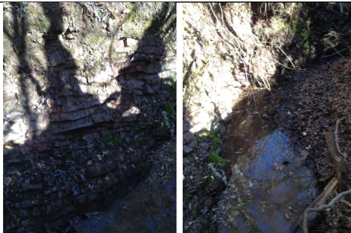
Photo 16. Taken approximately 520 ft upstream of the Live Oak culvert facing the right bank and upstream, respectively
