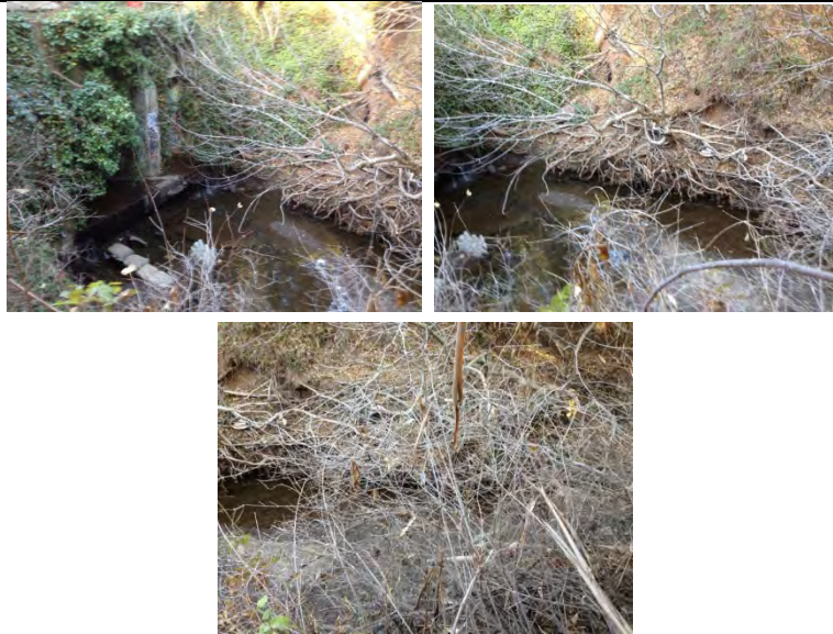
Photo 39. Taken downstream of the culvert outfall located east of 1301 Ralston Avenue, facing upstream, the left bank, and downstream, respectively
