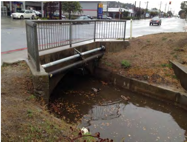
Photo 2. Old County Road Culvert
