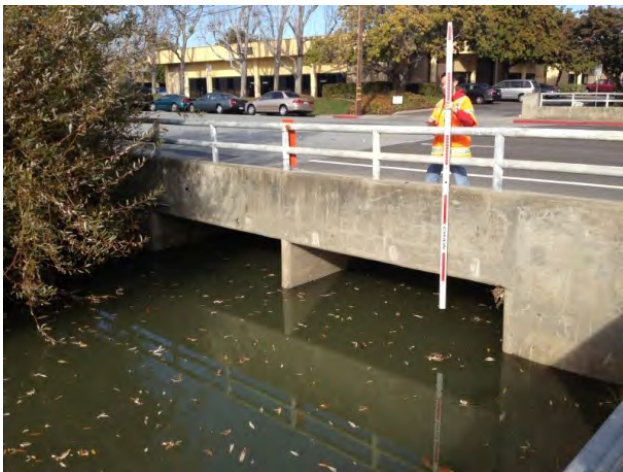
Photo 3. Industrial Road Culvert
