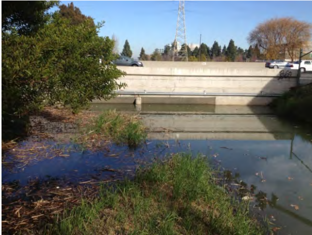
Photo 4. Old County Road Culvert
