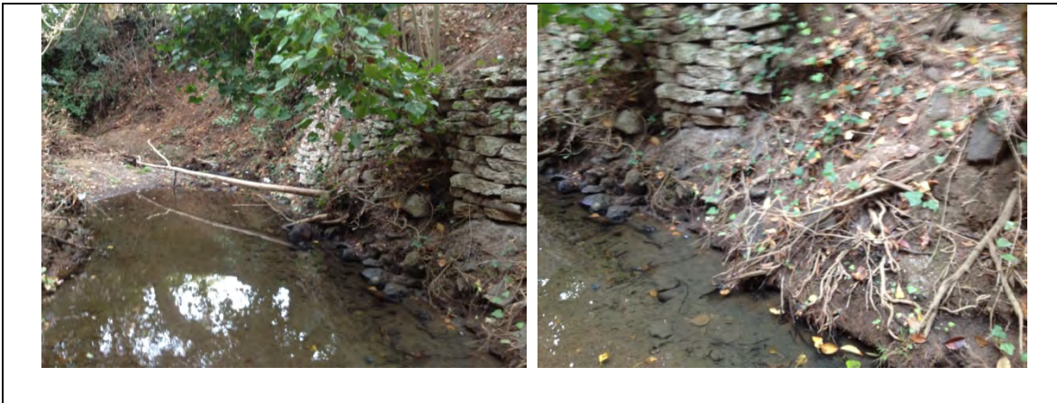
Photo 34. Taken approximately 600 ft upstream of the culvert crossing at Chula Vista Drive facing upstream and the left bank, respectively
