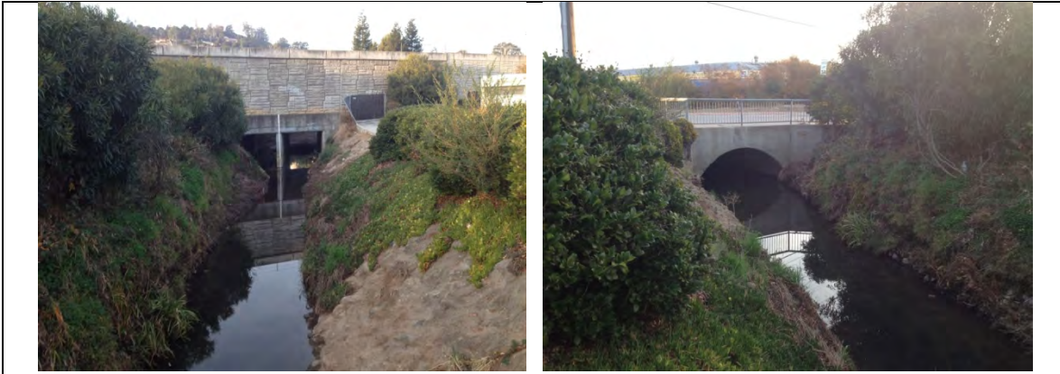
Photo 46. Taken between Old County Road and the Caltrain tracks facing upstream and downstream, respectively
