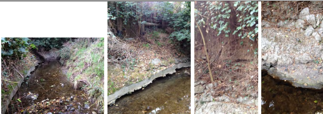
Photo 33. Taken approximately 700 ft upstream of the culvert crossing at Chula Vista Drive facing the upstream and the, respectively
