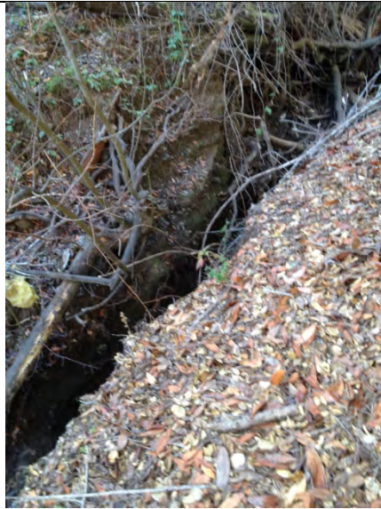
Photo 15. Taken approximately 520 ft upstream of the Live Oak culvert facing upstream
