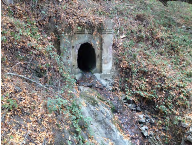
Photo 1. Water Dog Lake Outfall
