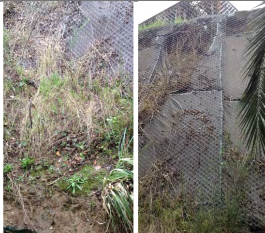
Photo 32. Taken approximately 870 ft upstream of the culvert crossing at Chula Vista Drive facing the left bank at the toe and top of bank, respectively
