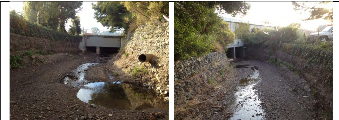
Photo 45. Taken from the culvert under the Caltrain tracks facing upstream and from El Camino Real facing downstream, respectively
