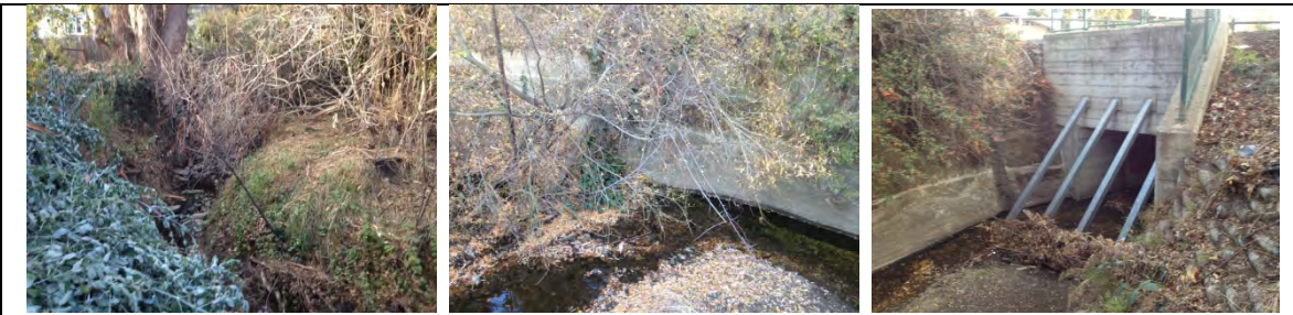
Photo 44. Taken between immediately southwest of 6th Avenue facing upstream, at a bend in the channel, and downstream at the reinforced concrete structure under 6th Avenue, respectively
