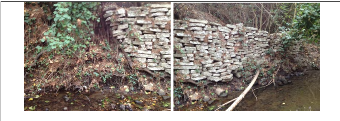
Photo 35. Taken approximately 530 ft upstream of the culvert crossing at Chula Vista Drive facing the right bank and right bank/upstream, respectively
