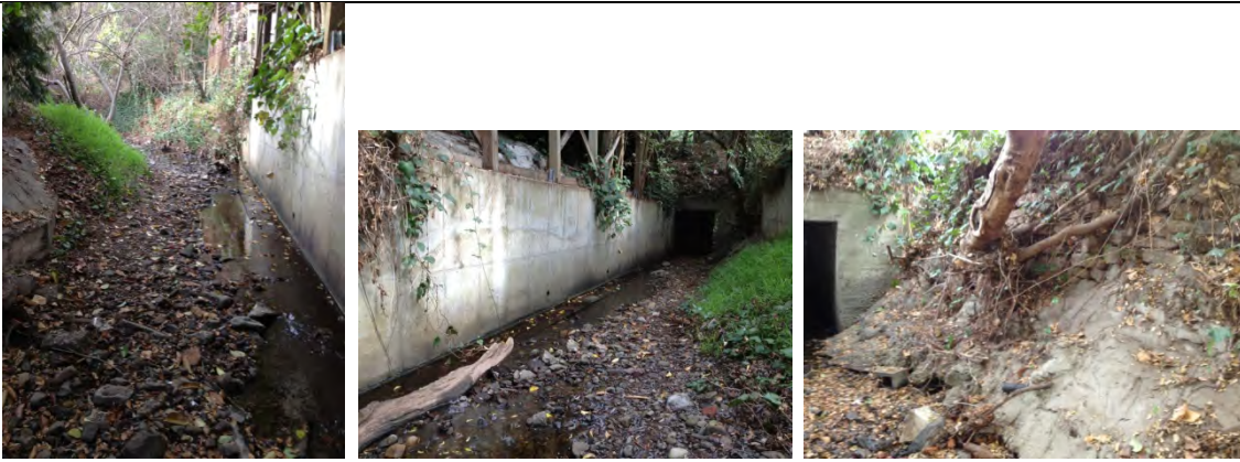
Photo 38. Taken at the upstream end of the culvert crossing under Chula Vista Drive facing upstream, downstream, and the right bank at the culvert, respectively
