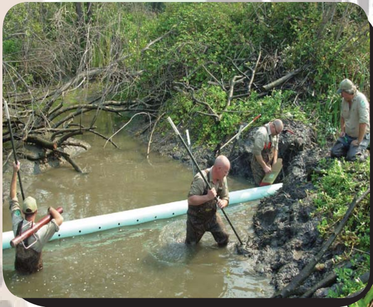
Technicians installing the Clemson Beaver Pond Leveler which is used to divert water through a pipe and lower the beaver pond to a manageable level.
