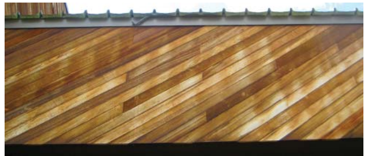
A-8 White Streaking Marks At New Team Room Soffit
