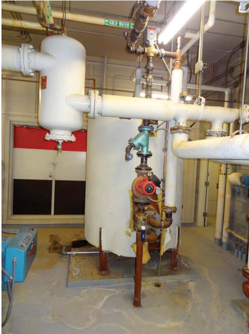
M-13 Domestic Water Tank Drain
