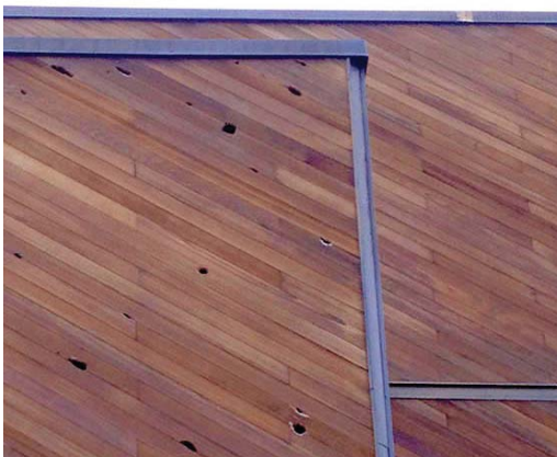
A-7 Bird Punctured Holes In Siding
