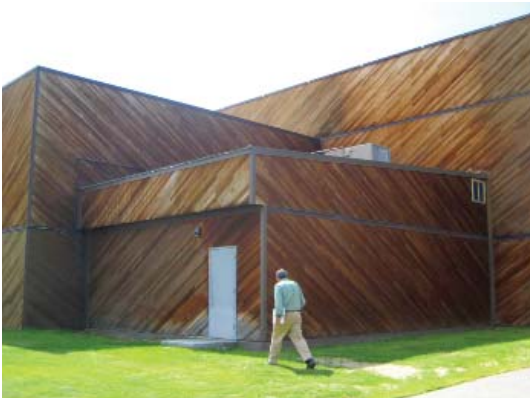
S-5 Wood Framed Locker Room Addition
