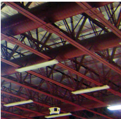
S-2 Steel Roof Joists
