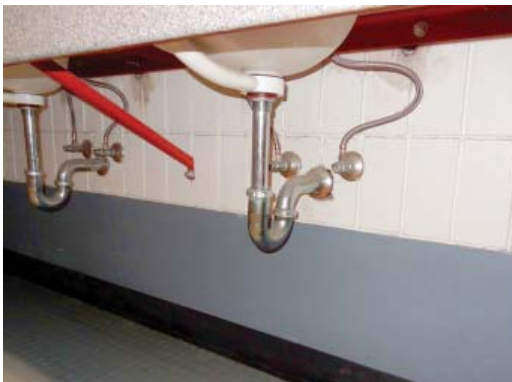
M-1- Uninsulated Waste, Hot Water
