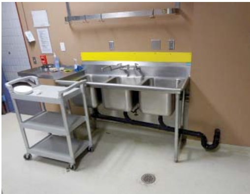
M-14 Three Compartment Sink, No Grease Interceptor
