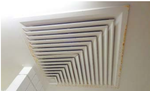
M-2.1 Grille Corrosion
