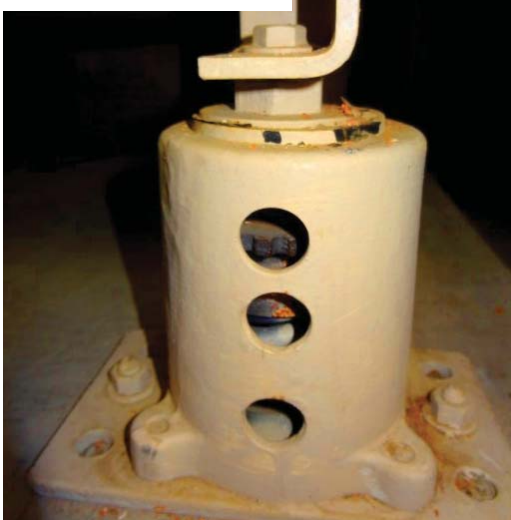
M-1 AHU-1 Bottomed out isolation
