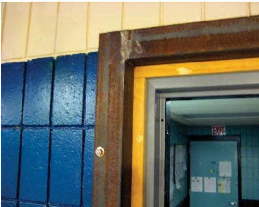
S-4 Doorway Cut Into Existing CMU Wall
