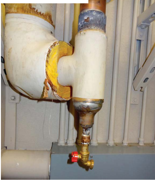
M-8 AHU-1 3-Way Valve Drain
