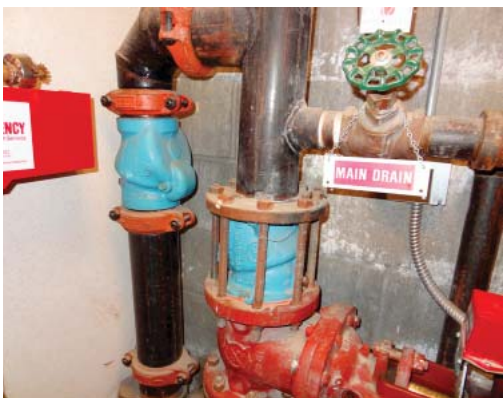
M-17 Sprinkler Check Valve
