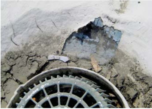
A-1 Roof Deterioration Around Drain
