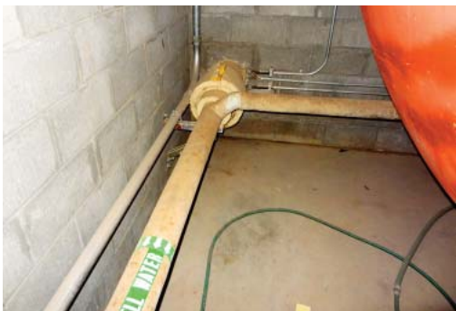
M-16 Undersized Sprinkler Line
