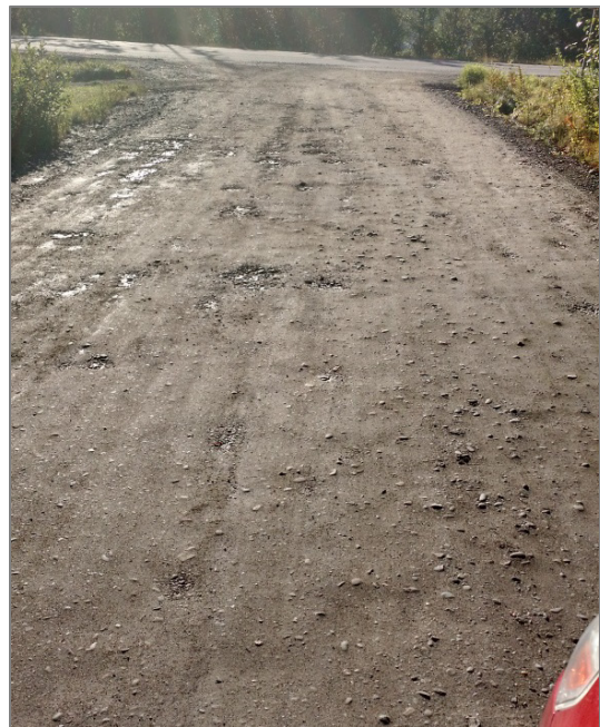
Figure 4 – Left: Gravel Road in Good Condition (Rating 8) / Right: Gravel Road in Poor Condition (Rating 4)
