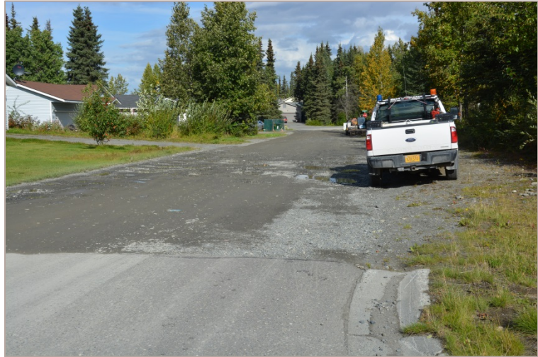
Figure 16 – Unpaved Segment of Lord Baranof Street
