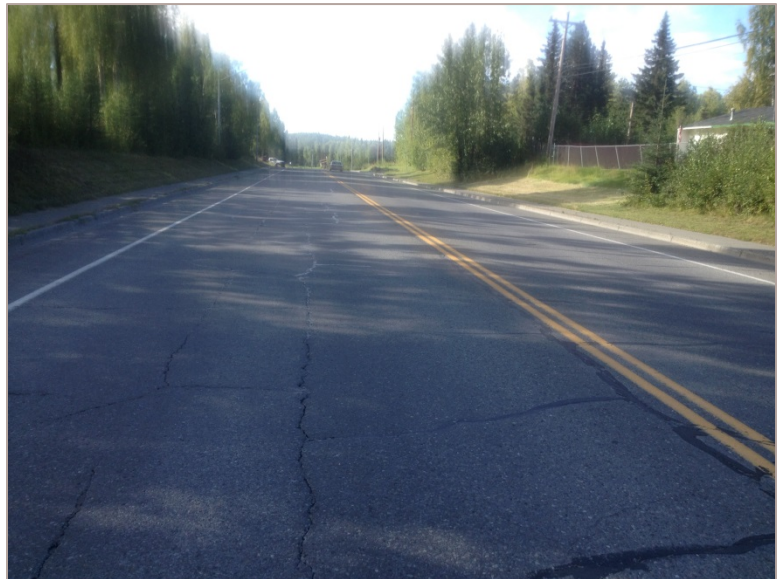
Figure 15 – South Kobuk Street
