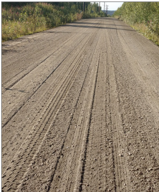
Figure 4 – Left: Gravel Road in Good Condition (Rating 8) / Right: Gravel Road in Poor Condition (Rating 4)
