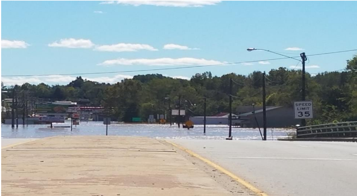
2018 flooding – view of Highway501 looking south in Riverdale
