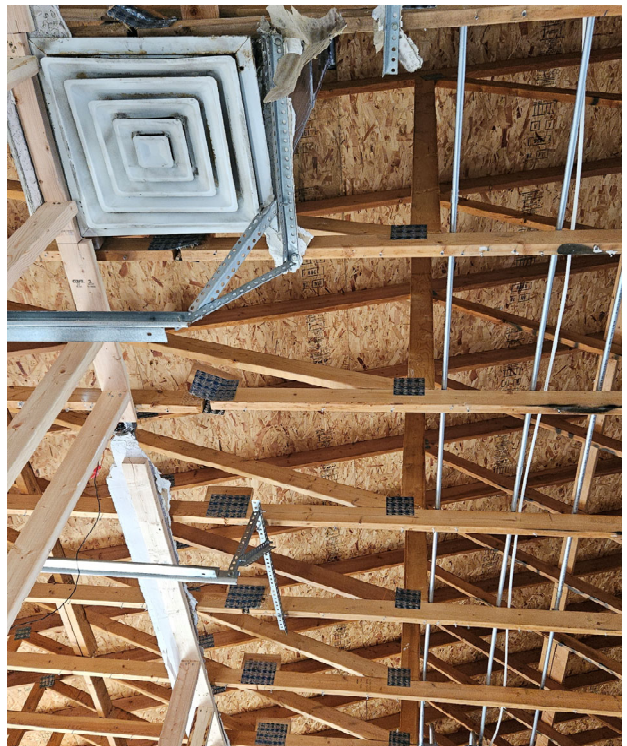
Line of Failed Bottom Chord Truss Plates
