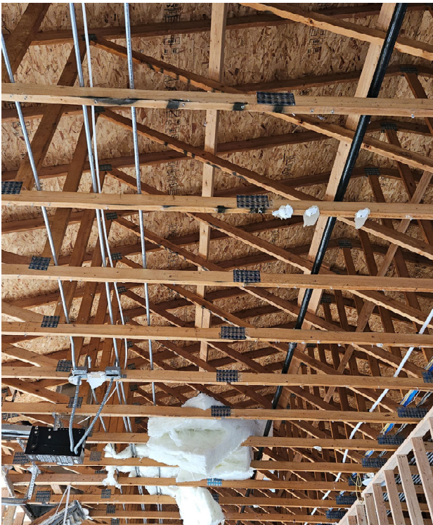
Line of Failed Bottom Chord Truss Plates
