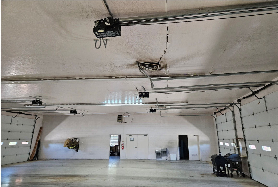
Interior Ceiling Crack @ East Third Point
