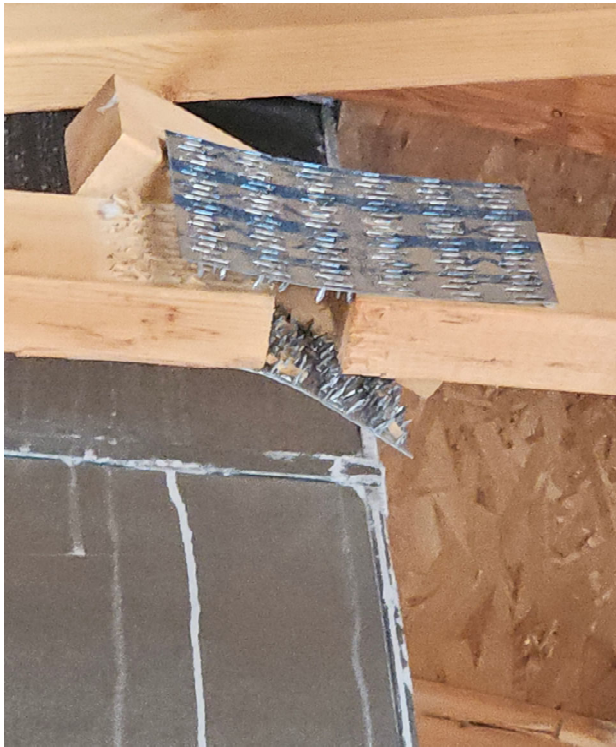
Failed East Third Point Bottom Truss Chord Plate
