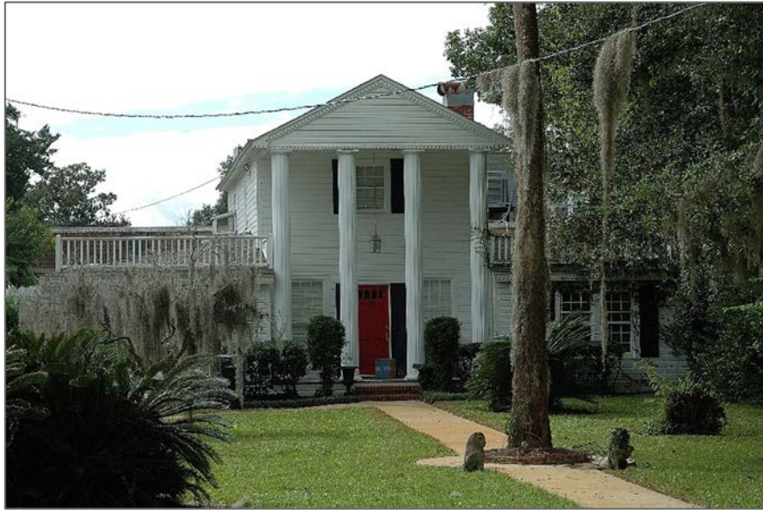
Figure 56. 102 E. Weed Street (c.1950), GNAHRGIS #281143 – This house is not representative of a building type identified by the Historic Preservation Division.
