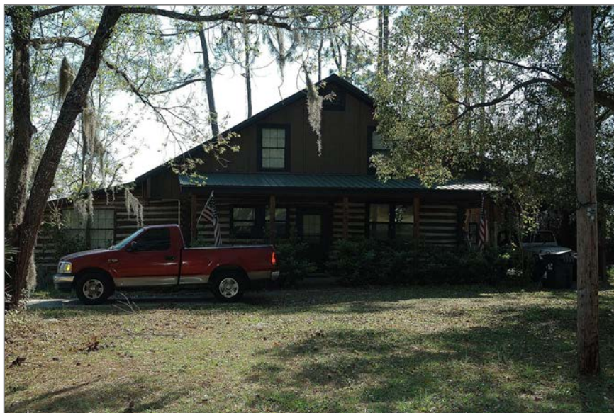
Figure 57. 508 Norris Street (c.1970), GNAHRGIS #283529 - This log, Adirondack style house does not appear to be representative of any academic building type.
