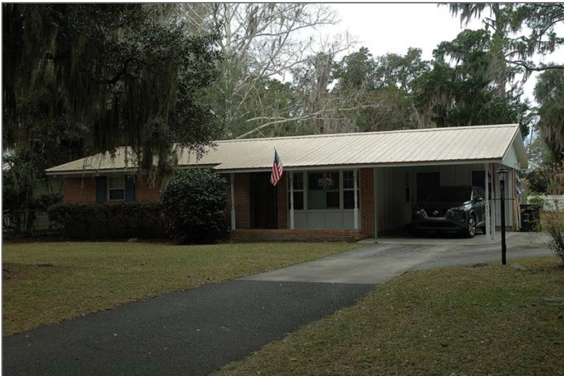
Figure 41. 407 Wheeler Street (c1967), GNAHRGIS #283183. Example of the compact ranch subtype - the length of the house is less than twice the width (minus the carport).
