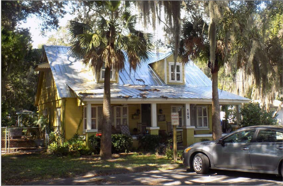
Figure 36. 105 Wheeler Street (c.1940) - GNAHRGIS #12586. Example of the side gable bungalow subtype.
