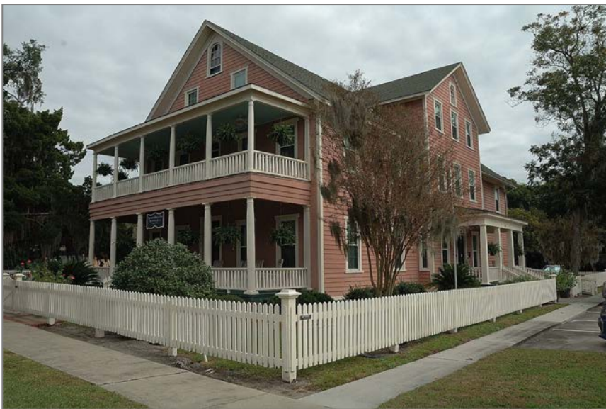
Figure 68. Long Hotel/Spencer House (c.1870), 101 E. Bryant Street, GNAHRGIS #12621. A typical late 19th century wood frame boarding house.
