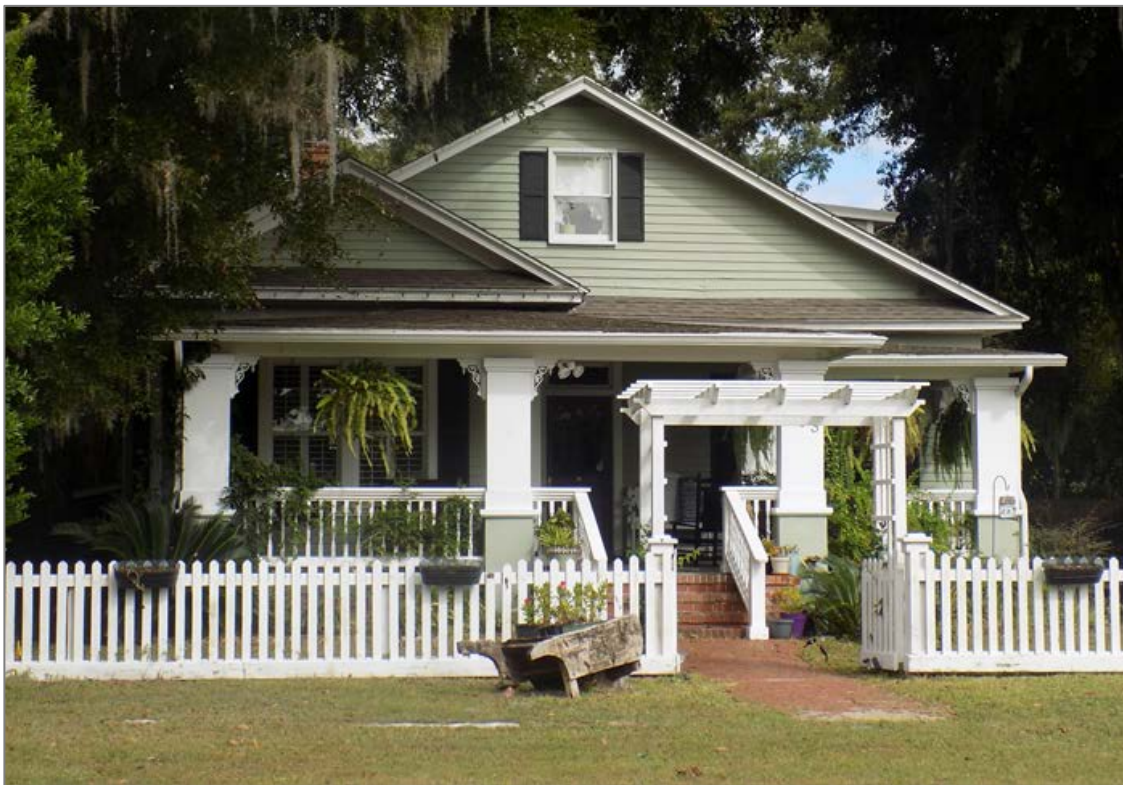
Figure 35. Smith-Aldridge House (c1919) - 103 E. Weed Street, GNAHRGIS #12633. Example of the front gable bungalow subtype.
