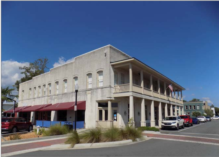
Figure 67. The Riverview Hotel (c.1916), 105 Osborne Street, GNAHRGIS #12578. A good example of a classic small town hotel.
