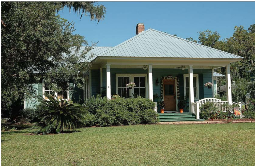
Figure 37. Townsend-Gay House (c.1905) - 202 W. Bryant Street, GNAHRGIS #12598. An example of the hip bungalow subtype.
