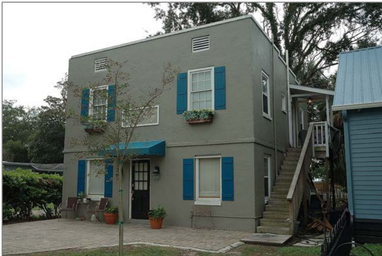
Figure 60. 102 E. Bryant Street (c.1950), GNAHRGIS #12620. An example of the duplex apartment type.
