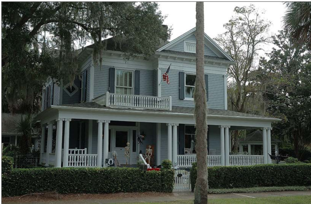
Figure 54. Bachlott-Porter House (c.1911), 220 Osbourne Street, GNAHRGIS #12625. An example of the Queen Anne house type as well as an excellent example of the Free Classic subtype of the Queen Anne style.
