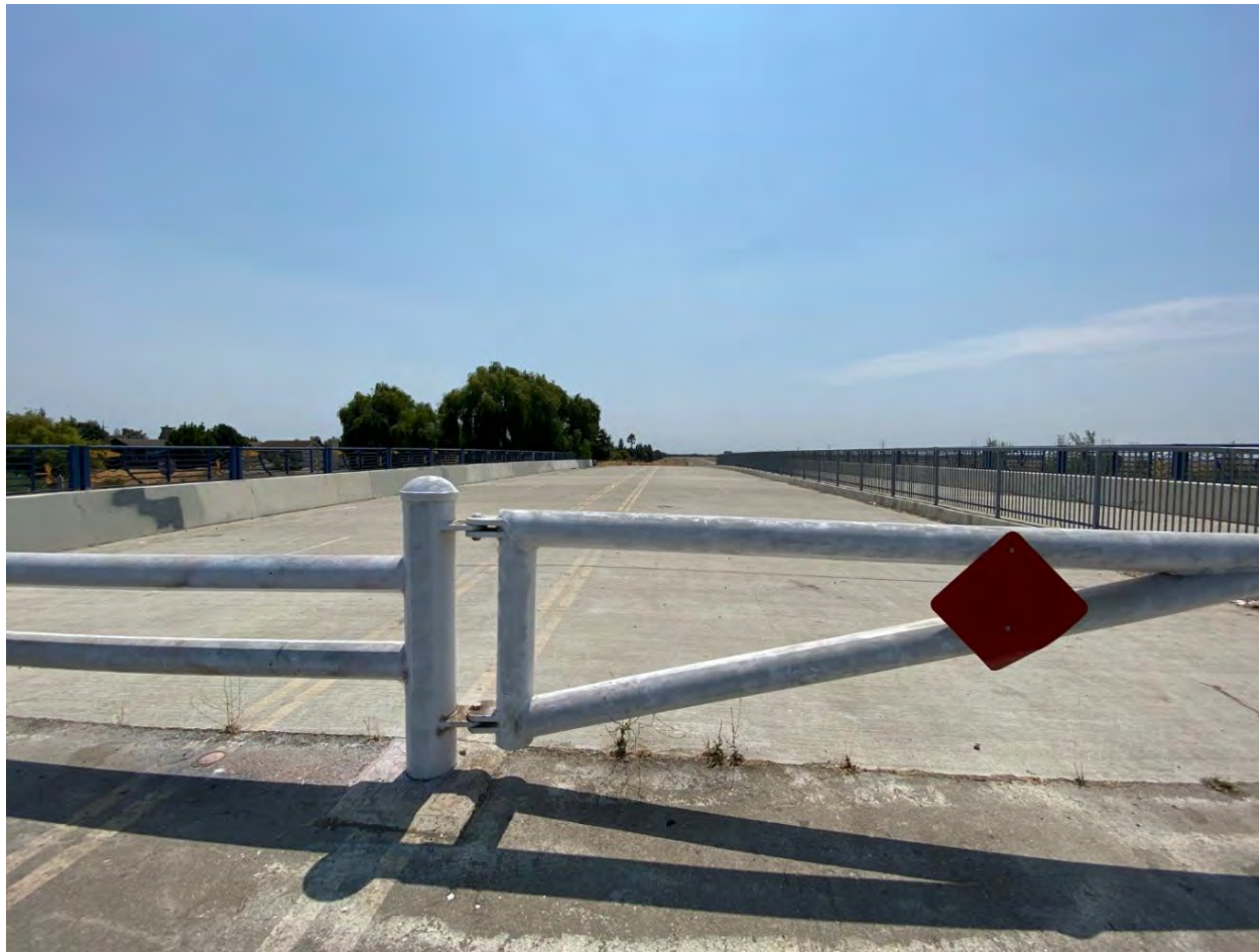
Trinity Parkway at end of bridge south of McAuliffe Road
