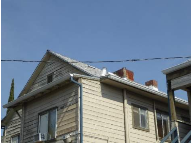
Figure 6. Aluminum slider windows, chimney, and ventilation pipes on roof above the southeast façade, view northeast.
