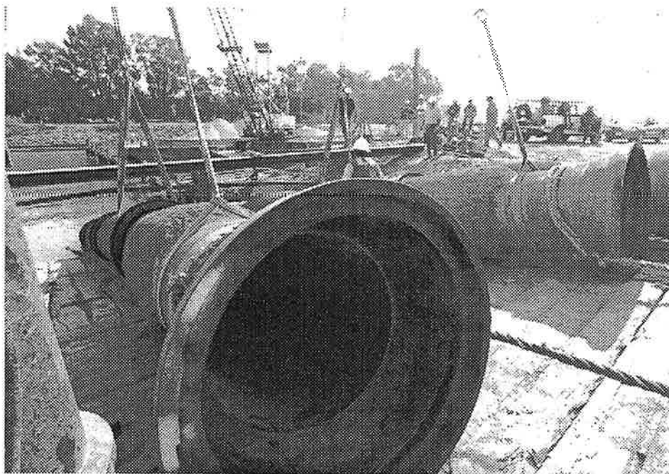
These 36-inch-diameter, iron sewer pipes are a part of the West Side Sewer Interceptor Project. The interceptor is an 8-mile long pipeline that will skirt levees on the City's west side to carry sewage from a pump station near Brookside Estates to the Navy Drive treatment plant. Photo courtesy of The Record.
