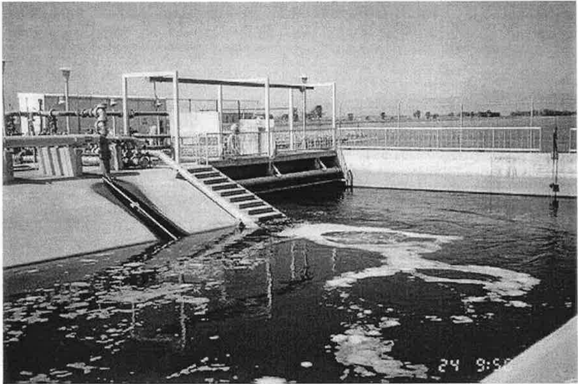
The Primary Sedimentation tank at the Municipal Utilities Treatment Plant.
