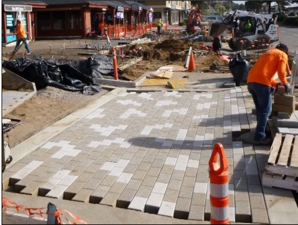
The installation of pavers at a crosswalk.
