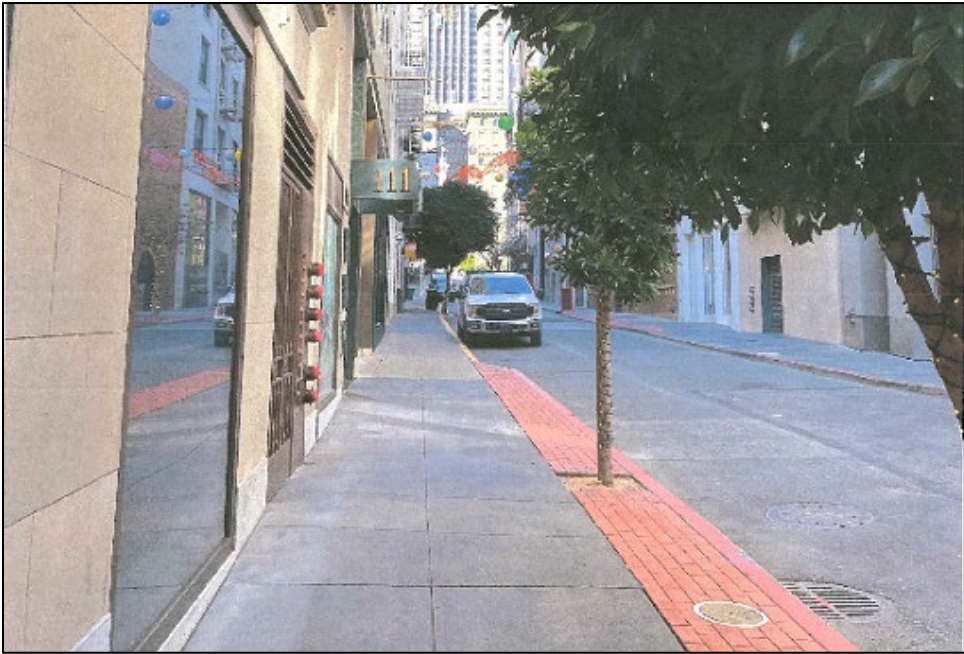
Level sidewalk for safer walking with pavers along street edge.
