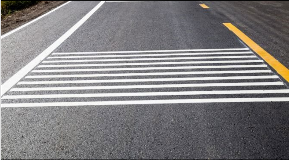
Rumble strips on the roadway.
