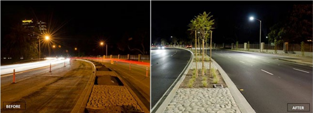
Improved nighttime visibility through LED lamp fixtures. Improves light uniformity, distribution and color rendering.
