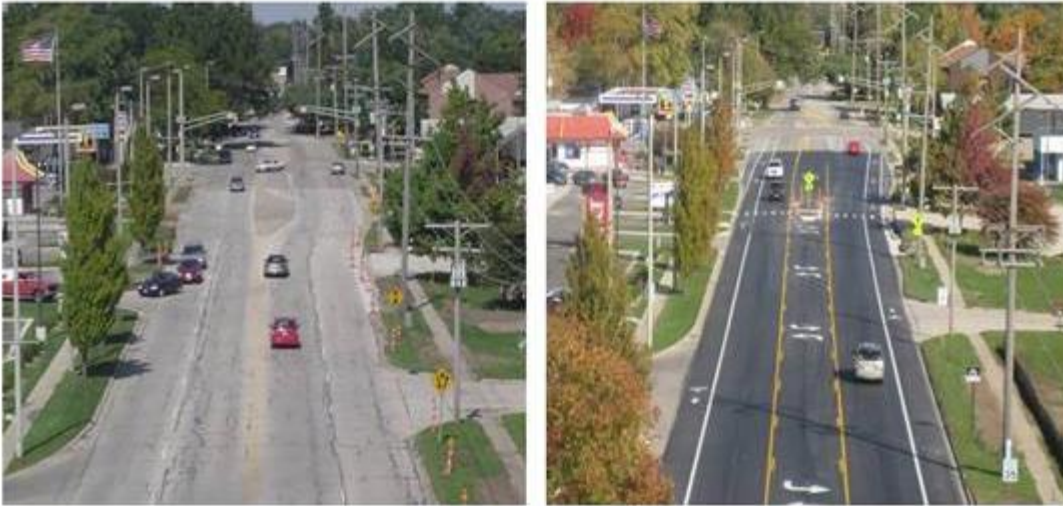
Figure 24: Example of Road Diet (Roadway Cross-Section Before and After Reconfiguration).
