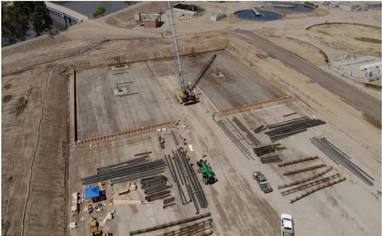
Aeration Basin looking west in May 2020.
