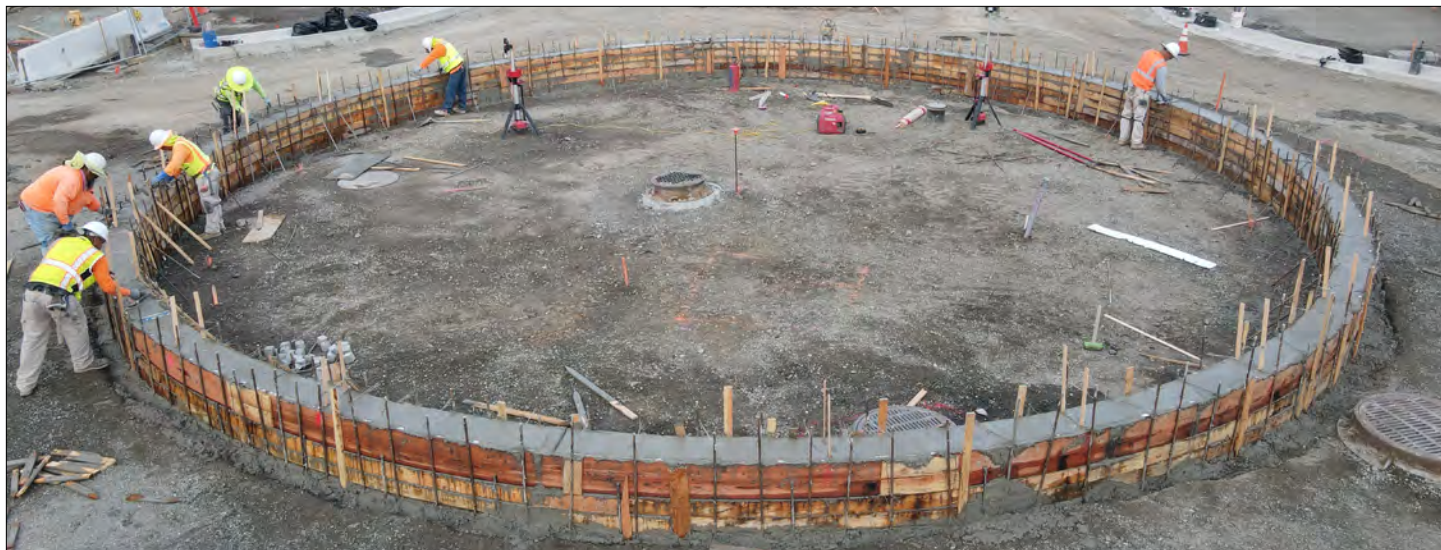
Construction workers pouring curbs at a roundabout at the intersection of San Joaquin and Miner, where TCC dollars are being used to make “complete street” improvements. Photo credit: City of Stockton
