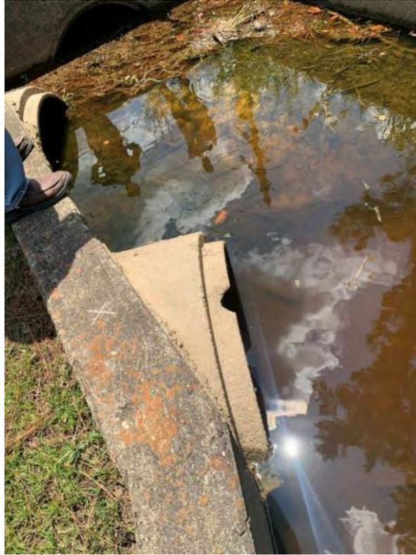
*Figure 28 - Inlet Box for Culverts on West Side Roadway Ditches and Driveway Culverts. Looking East.*
