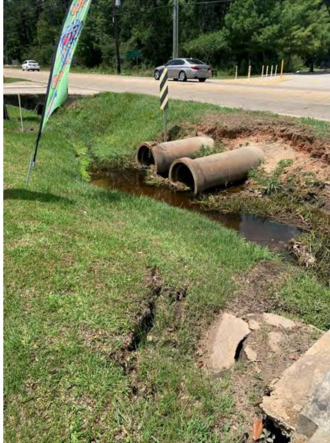
*Figure 19 - East Side Roadside Ditch and Cross Culverts along Highway 59. Looking Southeast.*
