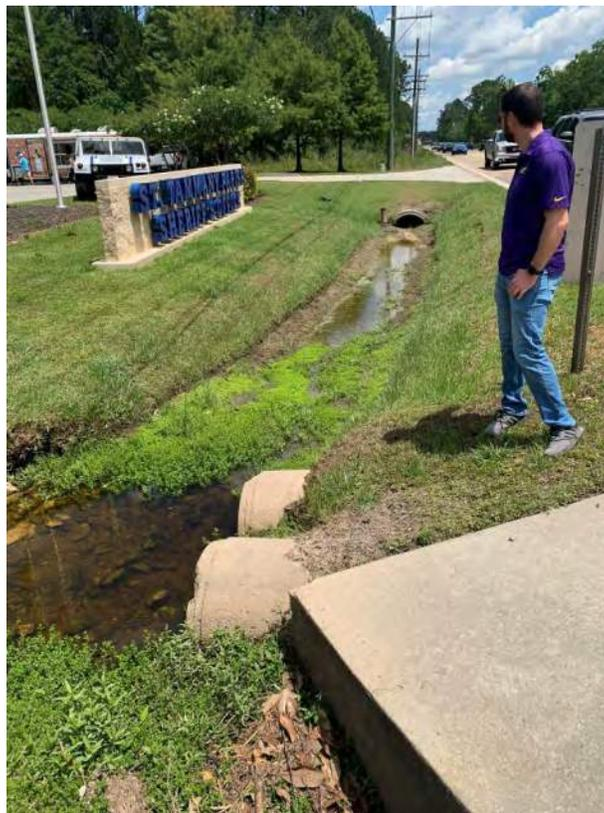
Figure 25 -West Side Roadside Ditch and Cross Culverts along Highway 59. Looking North.
