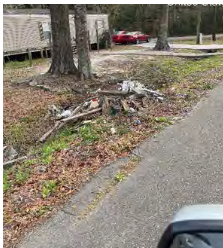
Figure 31 – Ditch filled with Debris
