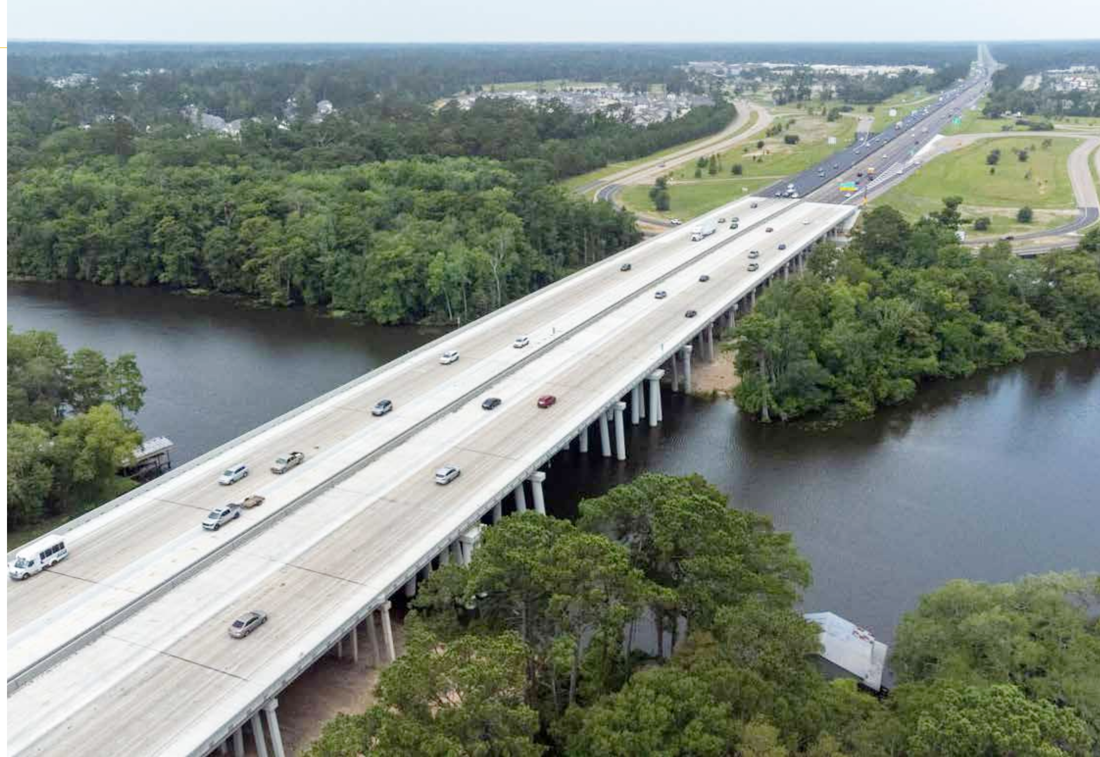
The newly widened Interstate 12 as seen over the Tchefuncte River near Covington.
