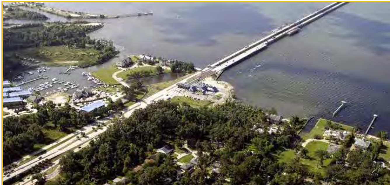
Lake Pontchartrain Causeway bridge and toll plaza.
