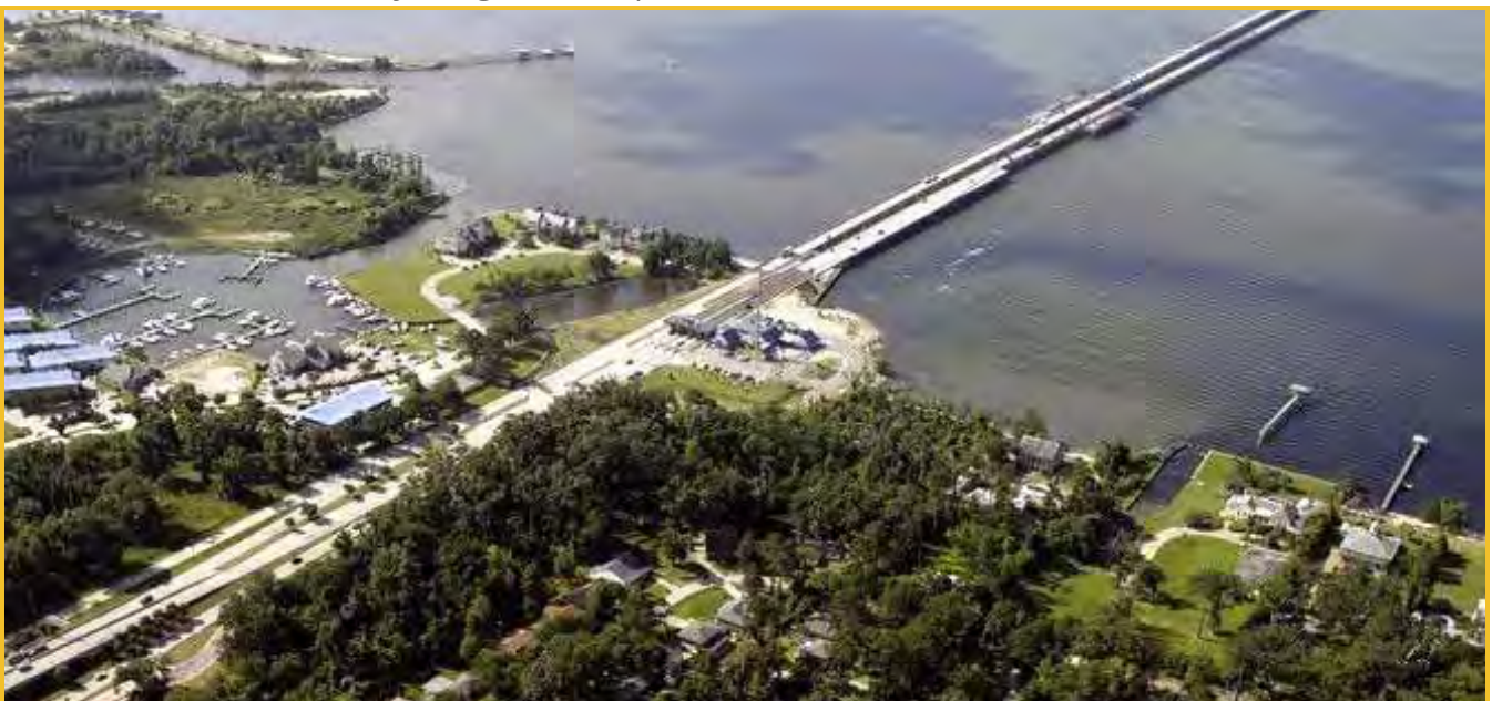
Lake Pontchartrain Causeway bridge and toll plaza.
