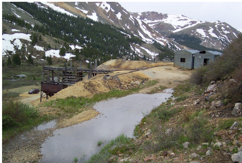
Standing water atop waste rock and mill tailings at Shoe Basin #1, 06/08/04
