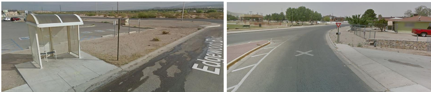
Figure 5-10 | Sidewalk Gaps within Sunland Park
