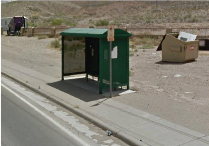
Figure 5-4 | Existing Bus Stop Amenities
