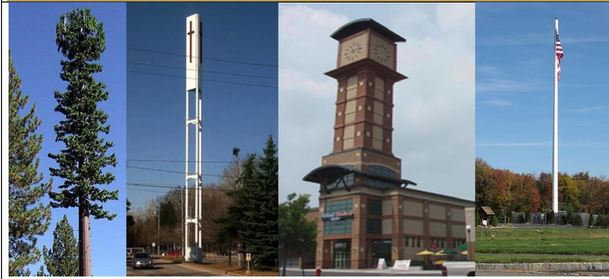
FIGURE 4.3.92, CONCEALED TELECOMMUNICATIONS FACILITIES
