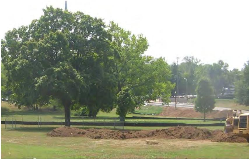
*The contractor installed chain-link fence around the “drip line” of the trees prior to construction.*
