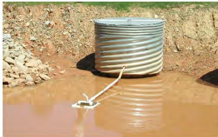
Figure 7.31-10B Floating Skimmer Installation
