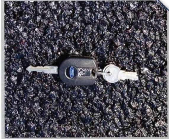
Close up of surface after Grip Tight Fog Seal
