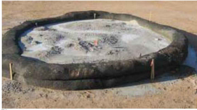
FIGURE 3.18 Typical Compost Sock Washout Installation
