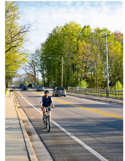
Figure 5-24. Example of a two-lane roadway with marked bicycle lanes Source: Wade Trim
