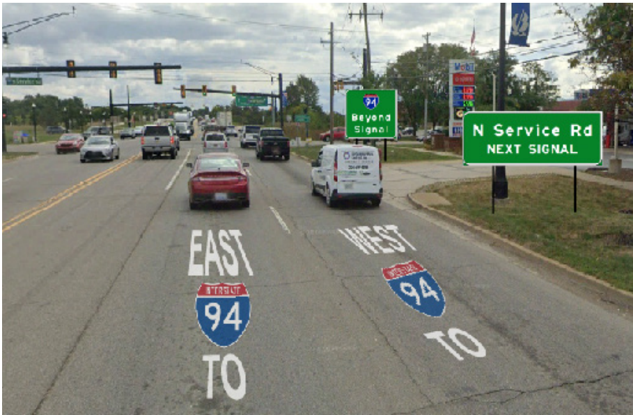
Figure 5-31. Installation of additional lane use and signage to provide clear direction Source: Wade Trim
