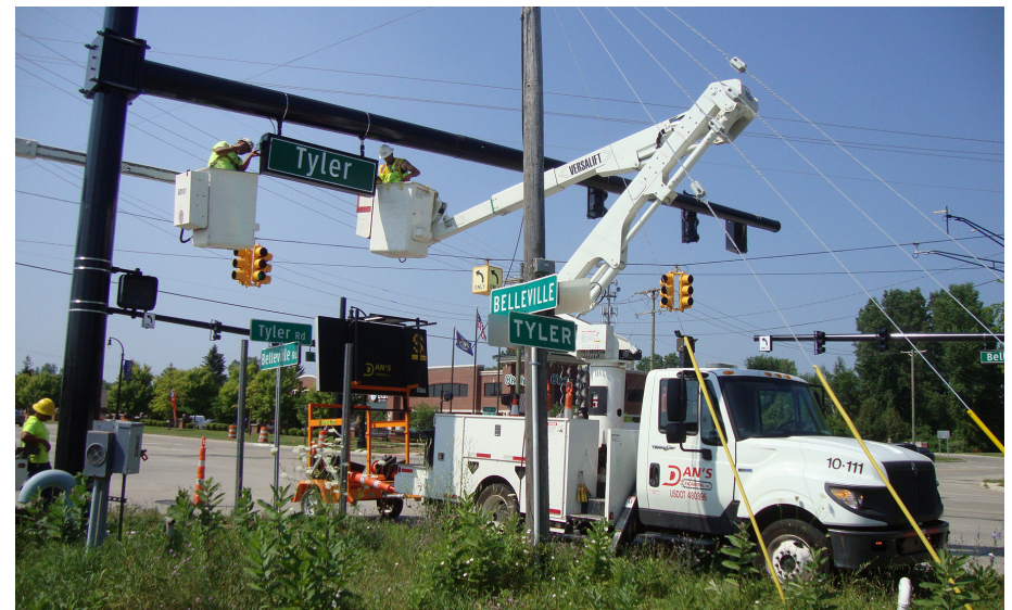
Figure 1-5. Signal upgrade project in Van Buren Township Source: Wade Trim
