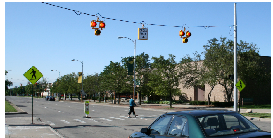
Figure 5-15. HAWK signal example
