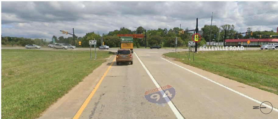
Figure 5-33. Installation of low level near side signals Source: Wade Trim
