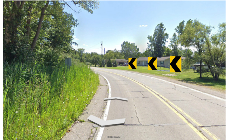
Figure 5-56. Haggerty Road & I-94 South Service Drive Source: Google Earth
