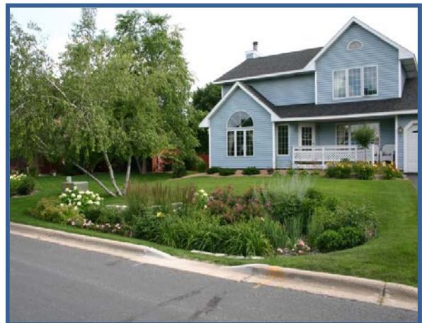
Figure C-10 An example of an LID practice which helps retain stormwater onsite while also providing filtration and pollutant removal benefits. (Photo courtesy of US EPA)
