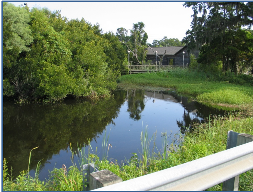
Figure H-13 An example of a vegetated stormwater pond in Murrells Inlet, which has been effective as reducing bacteria loads. (Photo courtesy of Murrells Inlet 2020)
