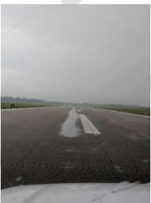
Figure 1: Potential Rutting left of Centerline - 2,000+ feet Southeast of Runway 11 end1
