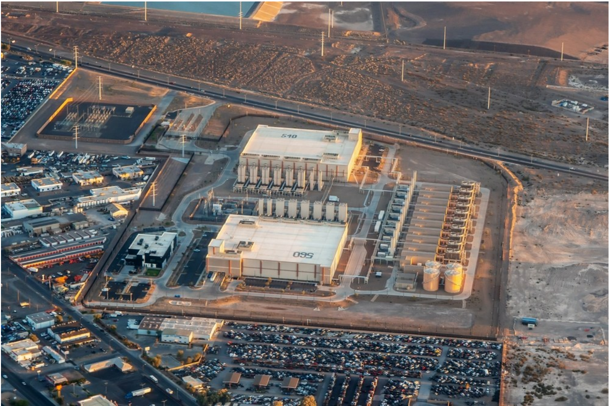
Aerial photo of a data center in Nevada. Image Credit: Audio und werbung/Shutterstock.com
