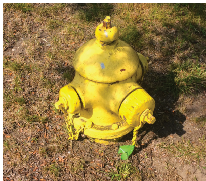
A tagged fire hydrant, indicating that it has been inspected and winterized.
