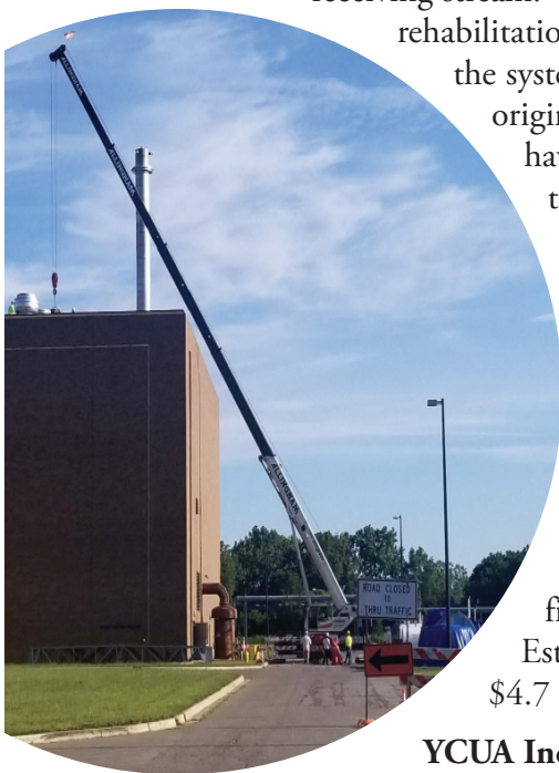
A crane at the YCUA WWTP removing the roof to allow access to the infrastructure below.
