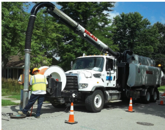
Vactors such as this are used by YCUA to clean about 65,000 feet of sewer mains each month.
