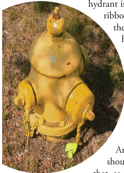
A tagged fire hydrant, indicating that it has been inspected and winterized.
