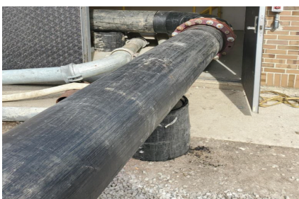
The 18-inch bypass pipe into the Snow Road wet well.
