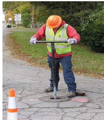
A YCUA employee conducting a valve turning exercise.
